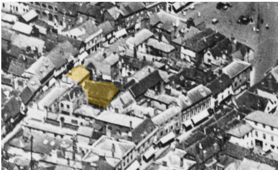
Fig.11: Aerial photograph taken 1925, property highlighted in yellow. A rear extension to the building formed with a pitched roof and two storeys high is visible. Though now reduced to single storey, evidence of the old roof can still be seen on the brick face.
