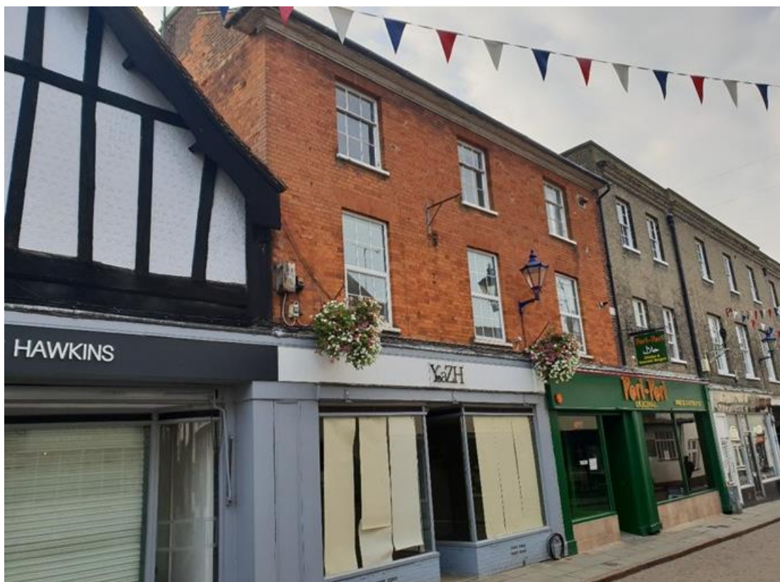
Fig.2: No.8 Bucklersbury is the last in the row of Hawkins buildings. No.7, visible on the left, is not the no.7 referred to in the listing description.
