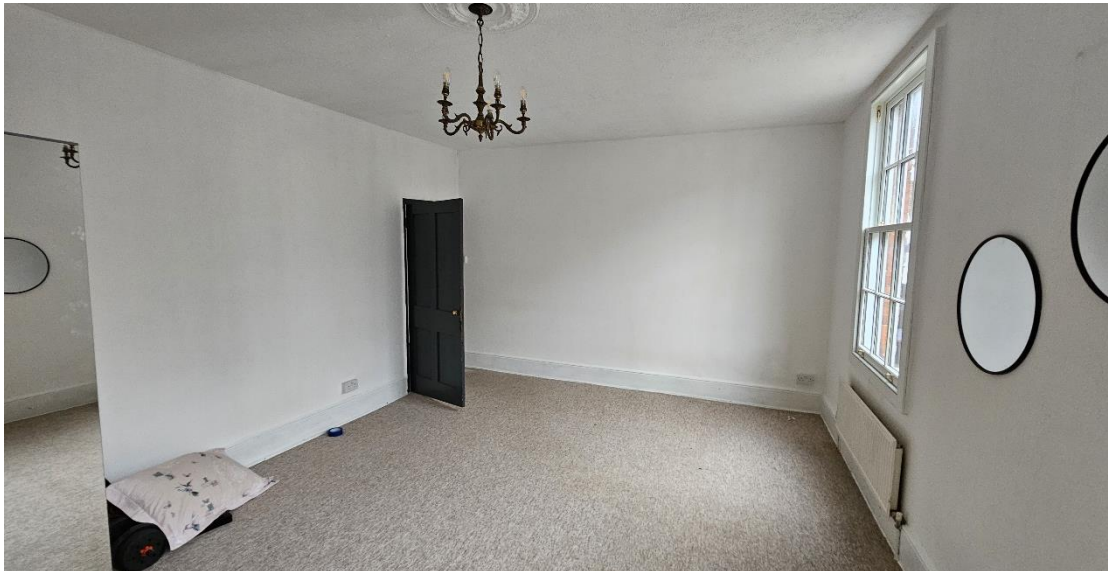
Fig.4: Large ground floor front room of the first floor, looking south.
