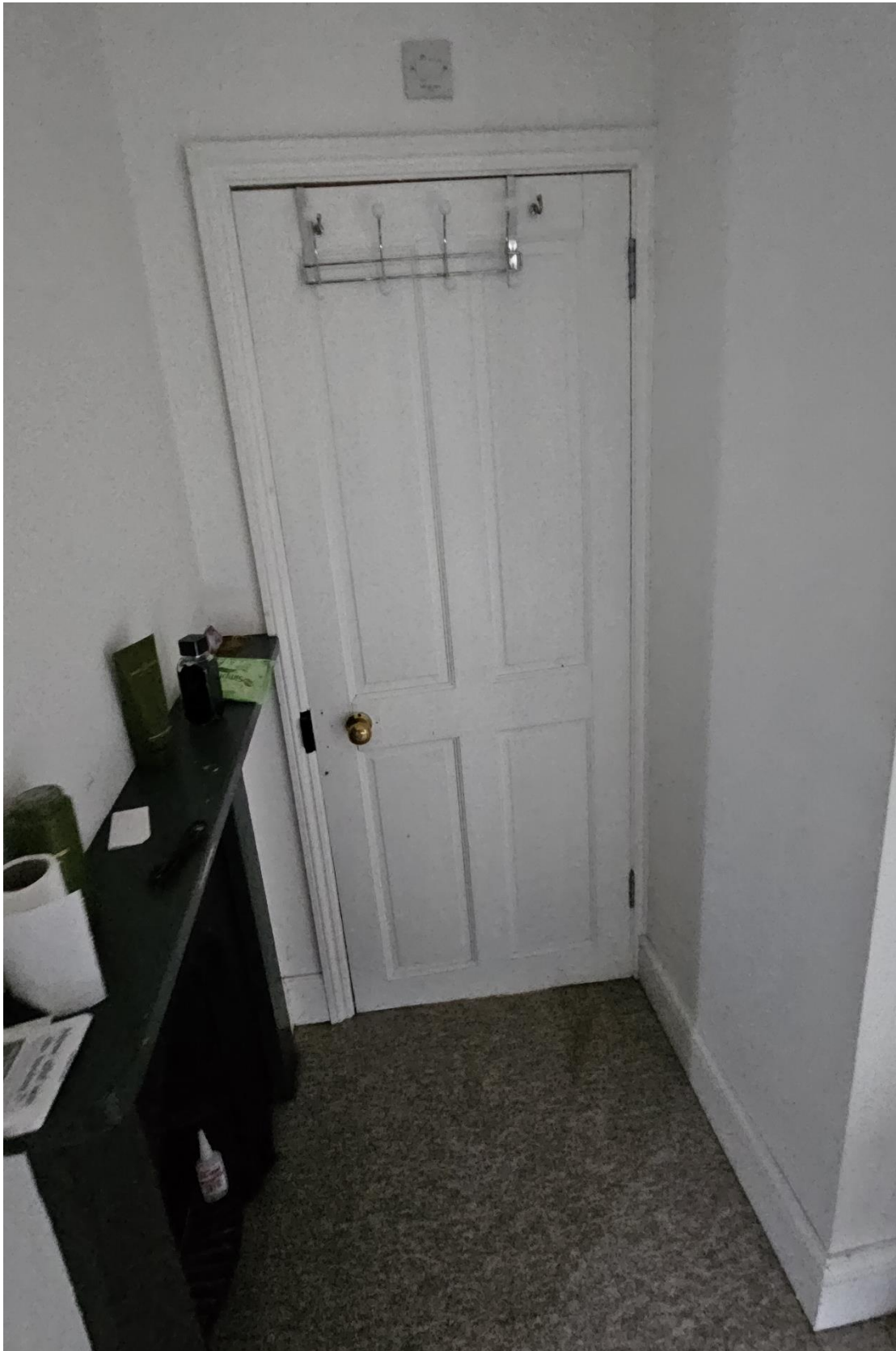
Fig.8: Post-construction door and partition adjacent to fireplace in the southern front room of the second floor.
