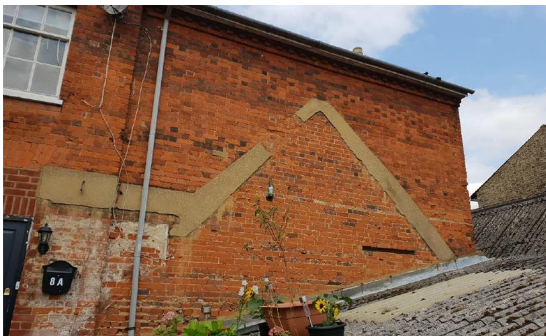
Fig.12: Rear (west) elevation showing cement render relating to a former extension attached to the building.
