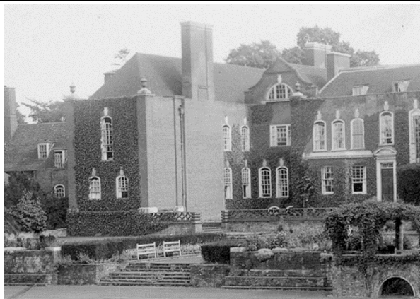
View of the East wing from the north prior to the roof being raised in 1935.
