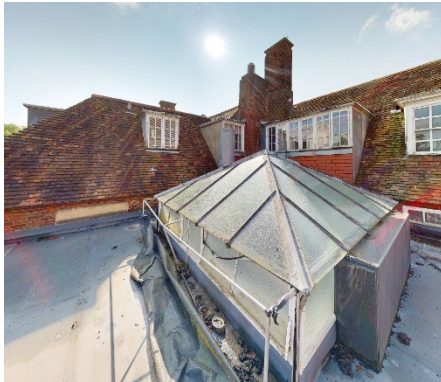
Present day photos of front and rear of level 1 of East Annex, south-east corner.
