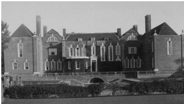
North rear elevation photo, post-Lutyens.
