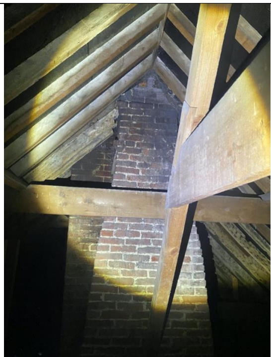
Central chimney inside loft space
