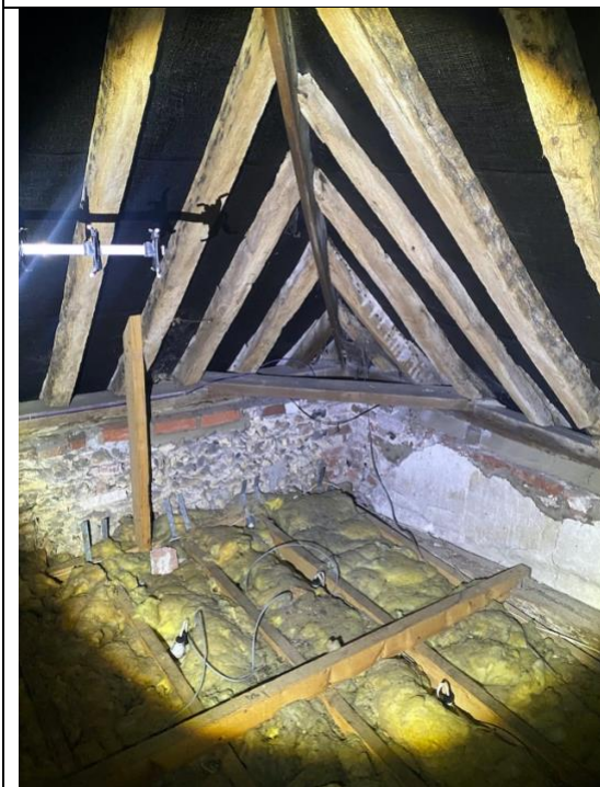
Timber rafters inside loft space.
