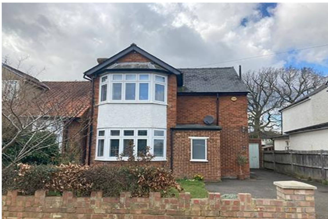
Above: View of front of 3 Old Hale Road from the highway
