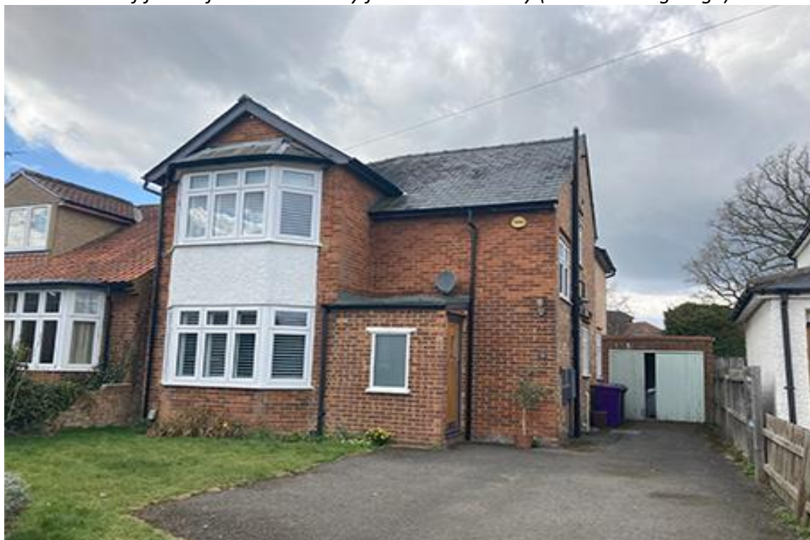
Below: View of front of 3 Old Hale Way from the driveway (to show the garage)
