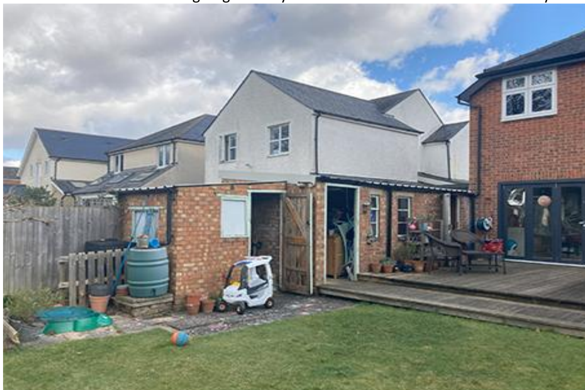
Photo below: View of existing single storey elements to the rear of 3 Old Hale Way
