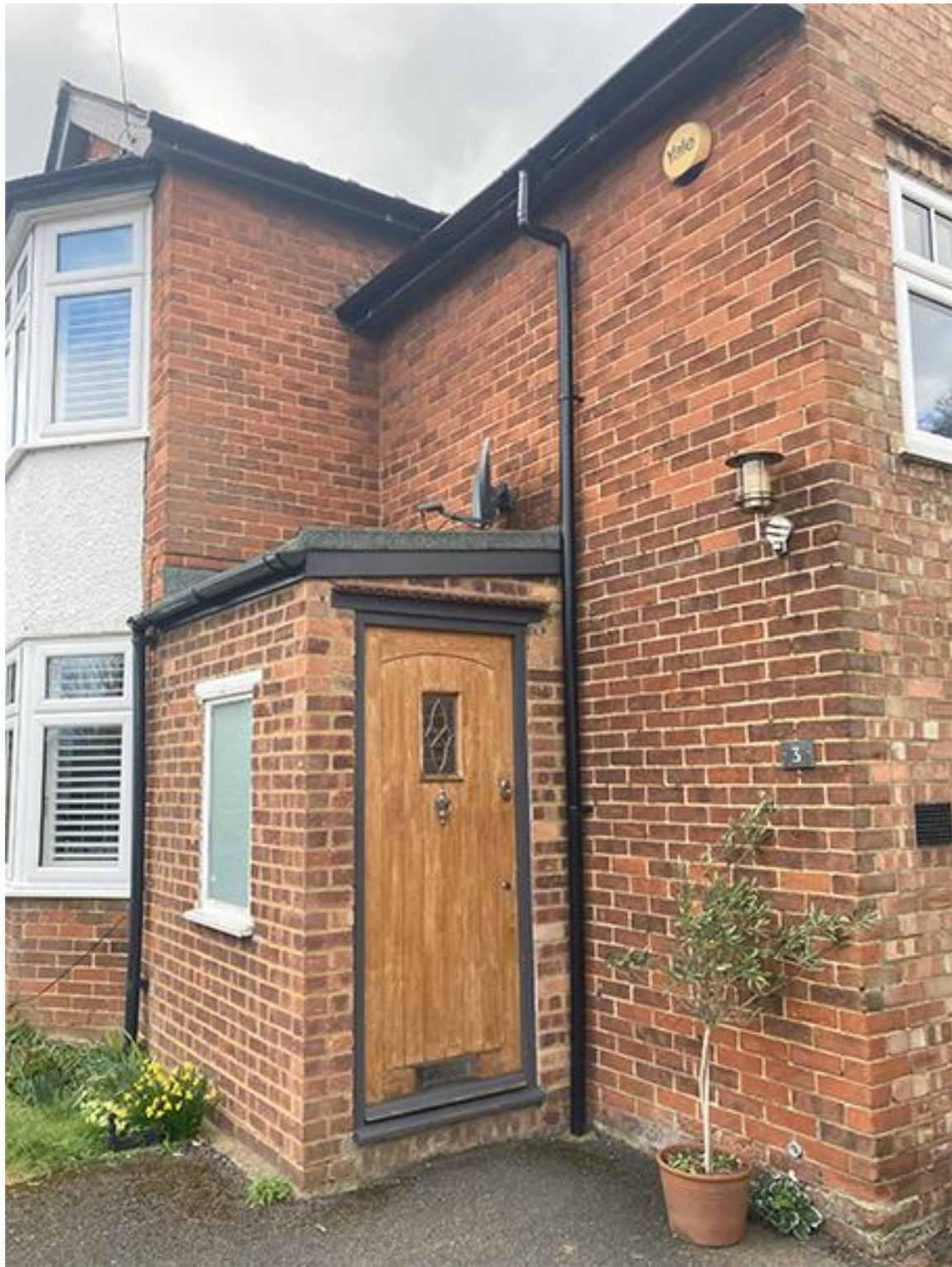
Photo above: View of existing porch at 3 Old Hale Way
