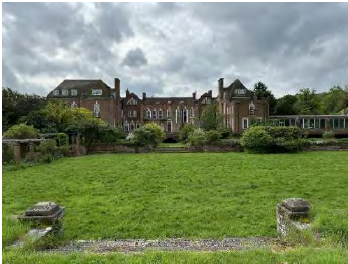
Figure 5: View of the lawn to the north of the main on-site building facing south-east.
