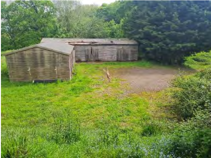
Figure 7: View of the timber clad stables to the north of the site facing north-east.
