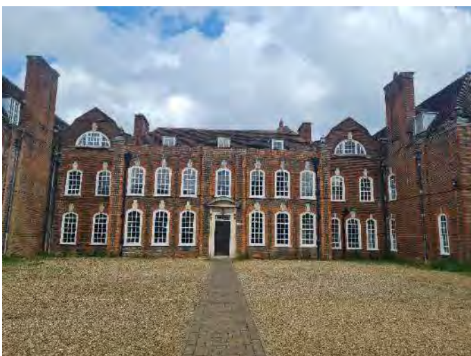
Figure 12: View of the main on-site building and gravel courtyard facing north-west.
