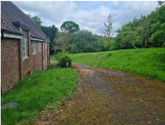
Figure 8: View of the asphalt track on the eastern boundary of the site facing north-west.
