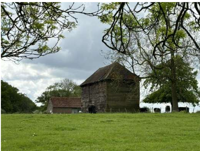
Figure 3: View of the timber clad barn in the north-western section of the site.
