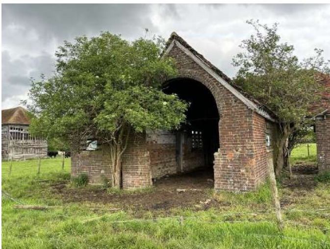
Figure 6: View of the pumping station facing north.
