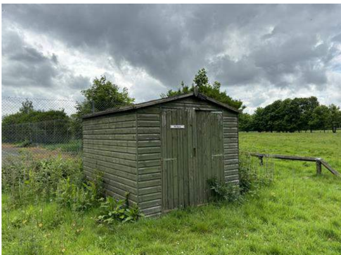
Figure 3: View of the small PE storage shed facing south-west.
