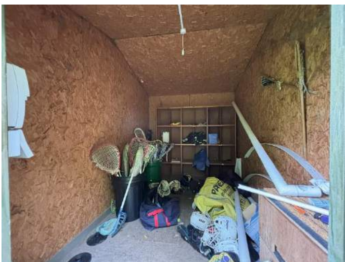
Figure 6: View of the PE equipment stored in one room of the outbuilding.
