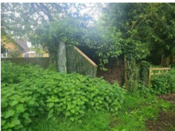
Figure 3: Outbuilding on the western boundary of the site facing south-west.
