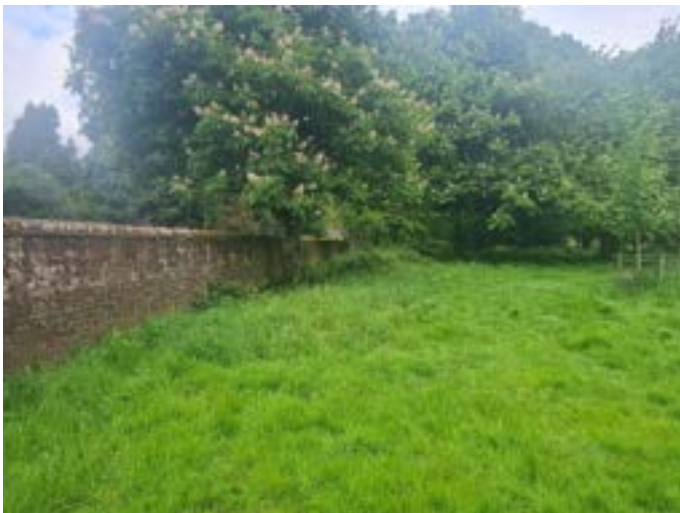
Figure 2: View down the south-western site boundary facing north-west.
