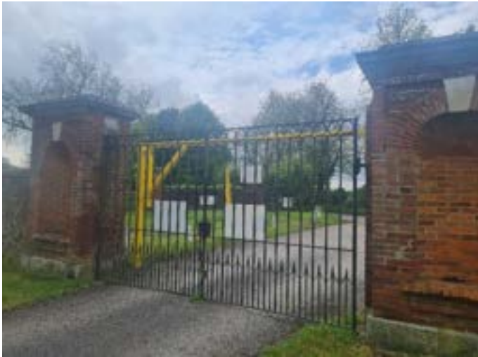
Figure 1: View of the site entrance facing south-east leading to a private driveway associated with Temple Dinsley.
