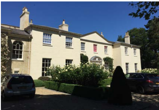
Fig 8. The east (entrance) front of the main range
