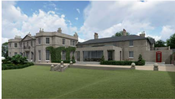
View of West Elevation
