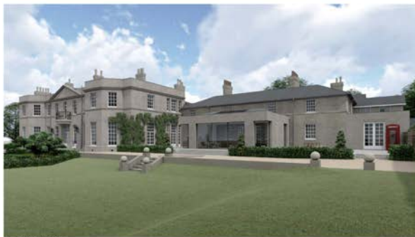
View of West Elevation
