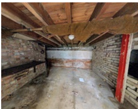
Modern fabric Stable block basement
