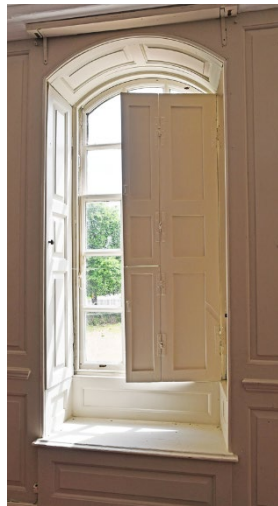
Windows and shutters
