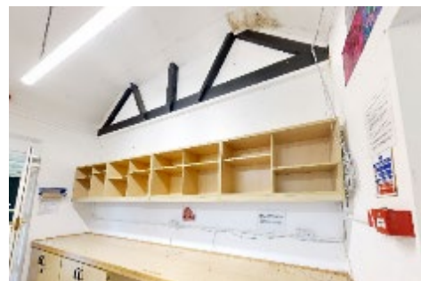
Interior of reused C19 building
