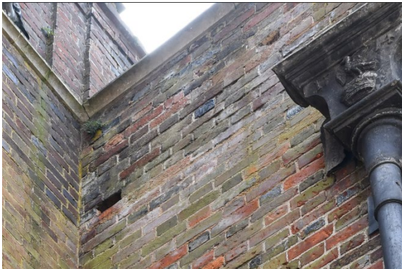
Water damage to parapet and brickwork
