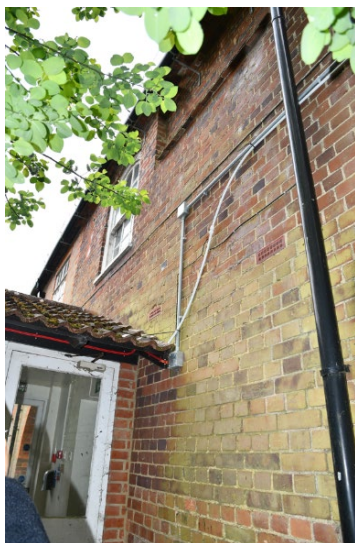
Rear with reused sash window
