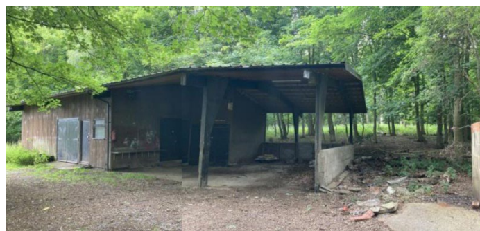
View on the approach to the Summerhouse within a clearing in the woods.
