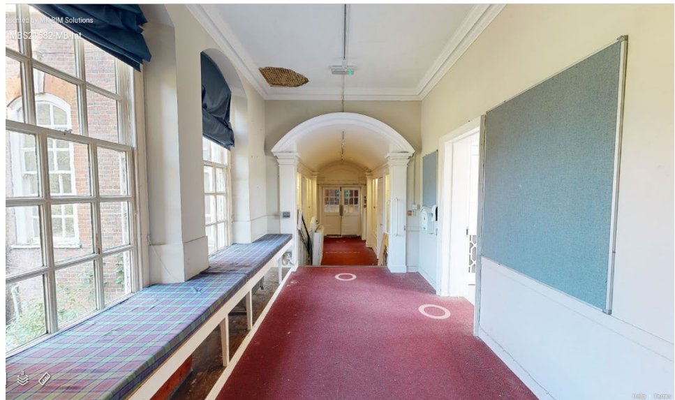
Service Corridor with some joinery including upper cornice, windows, arch and door surrounds by Lutyens.
