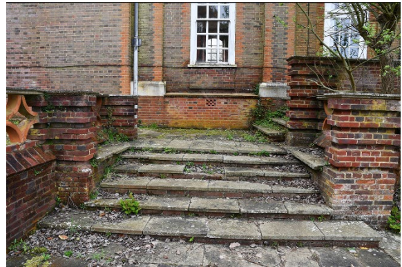
Damage to paving and external brickwork
