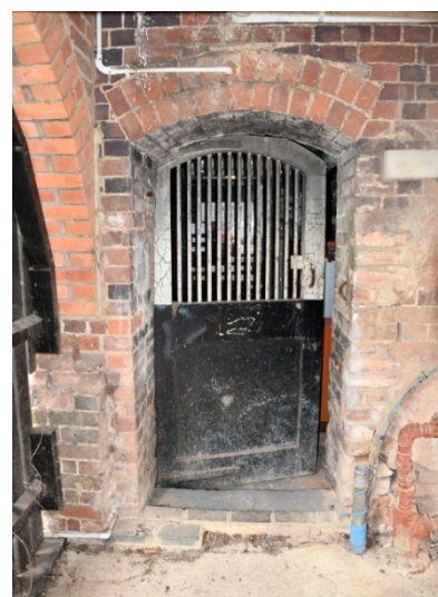
Door to Plant Room
