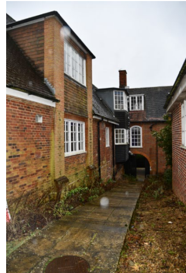
East Side with base of C19 wall
