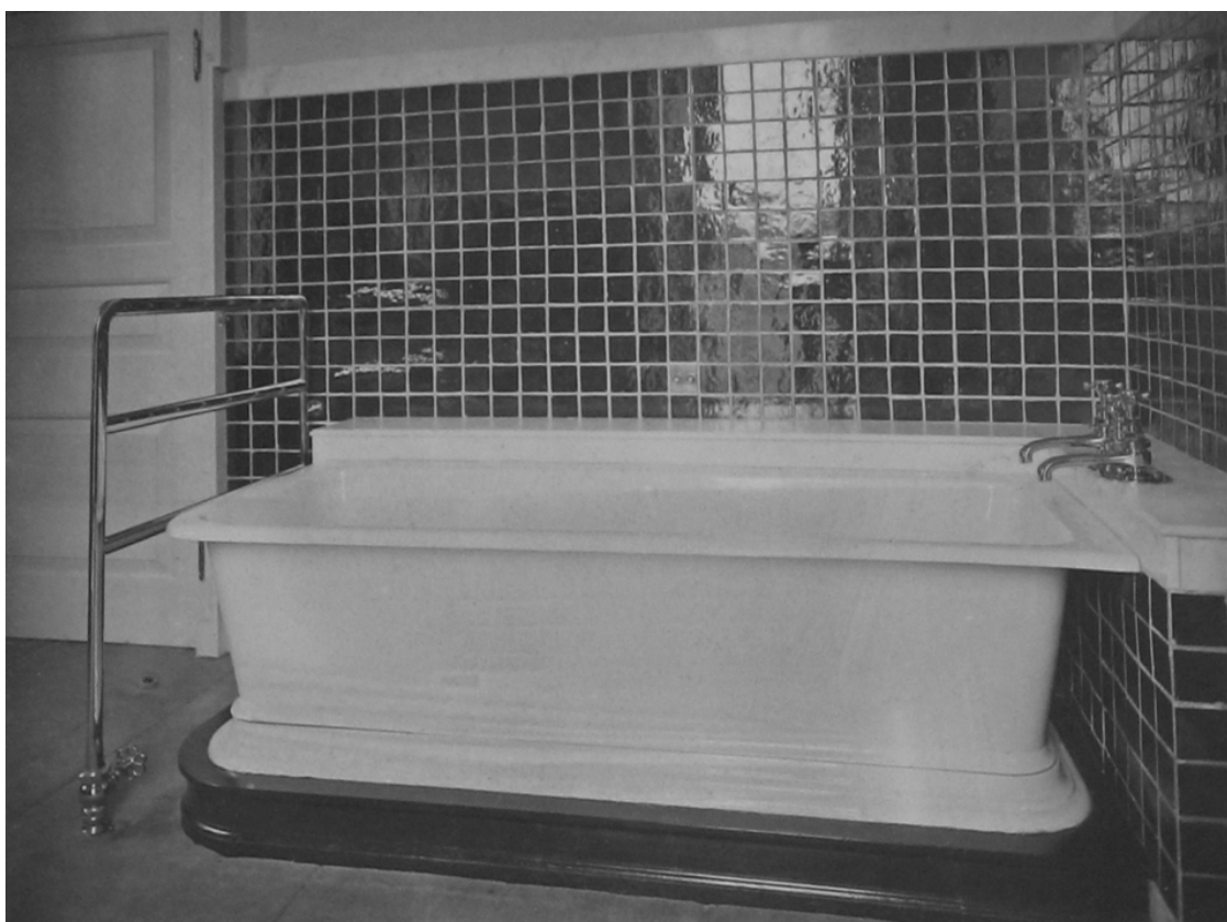
Bathroom First Floor West Wing North end. Country Life Collection.
