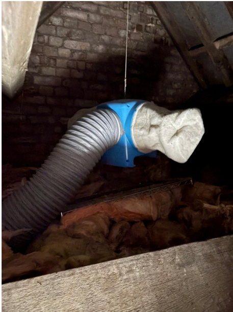
Picture 6 and 7 – Unventilated roof void, redundant positive air pump, and lowered eaves sections.
