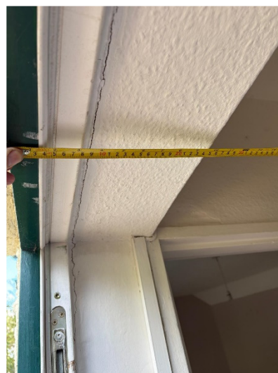
Picture 2 – Wall thickness demonstrated.
