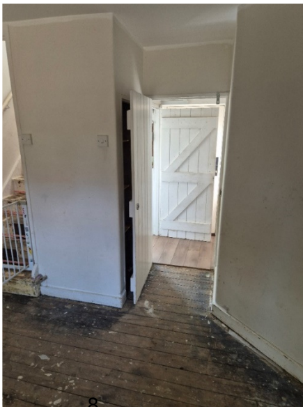
Picture 6, 7 and 7 – Juxtapose of differing floor finishes evidence of silver fish above solid floor construction and lack of air bricks evidenced to the rear elevation.
