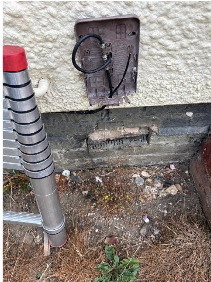
Picture 3, 4 and 5 – Floor Depth, front elevation damage air brick and clearly ventilated void. With
