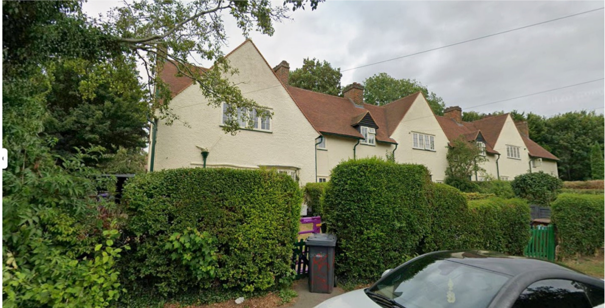
Picture 1 - Row of terraces representing the application, number 94 is the third gable roofed element of the building to the right of the picture.
