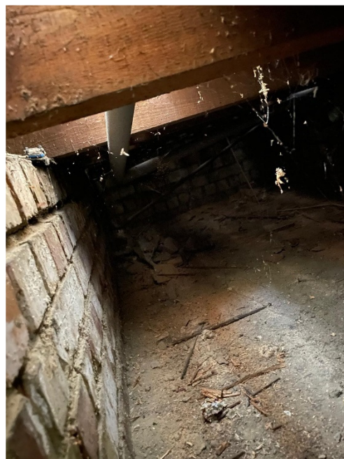
Picture 3 and 4 – Ventilation and clearly ventilated void.
