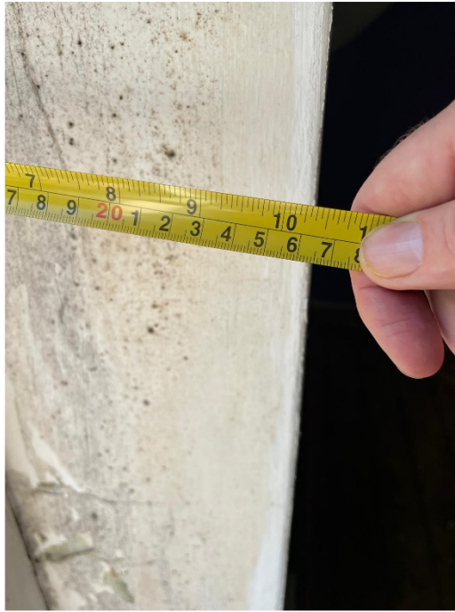
Picture 2 – Wall thickness demonstrated.
