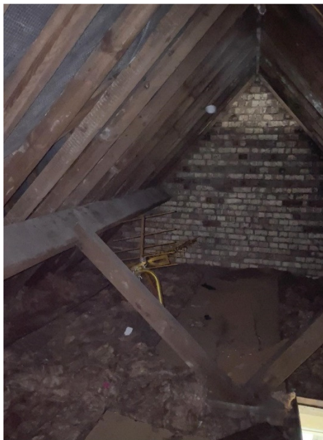
Picture 6 and 7 – Unventilated roof void, and lowered eaves sections.
