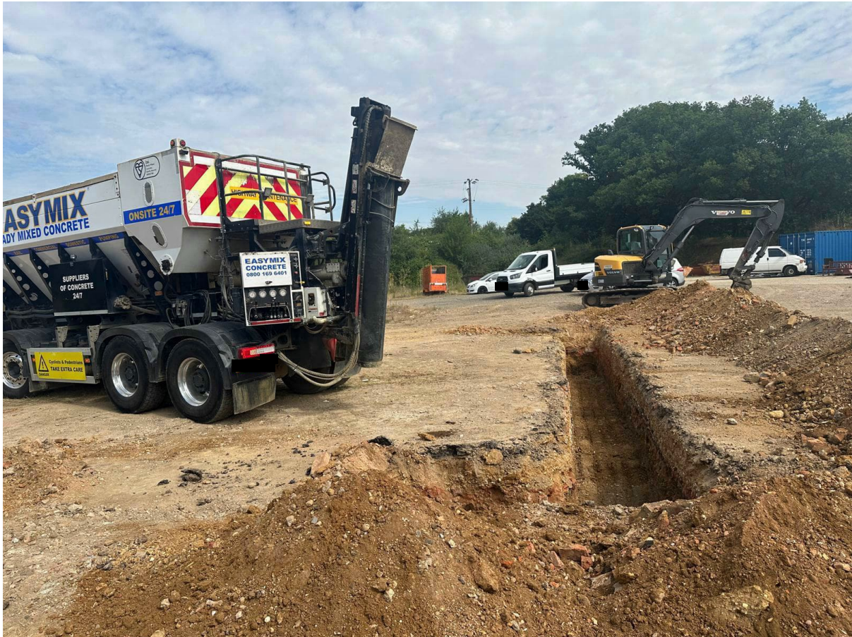
21/01535/F - Vicars Grove Pit, Little Almshoe Road, St Ippolyts, Hertfordshire: Evidence of a Material Start on Site
