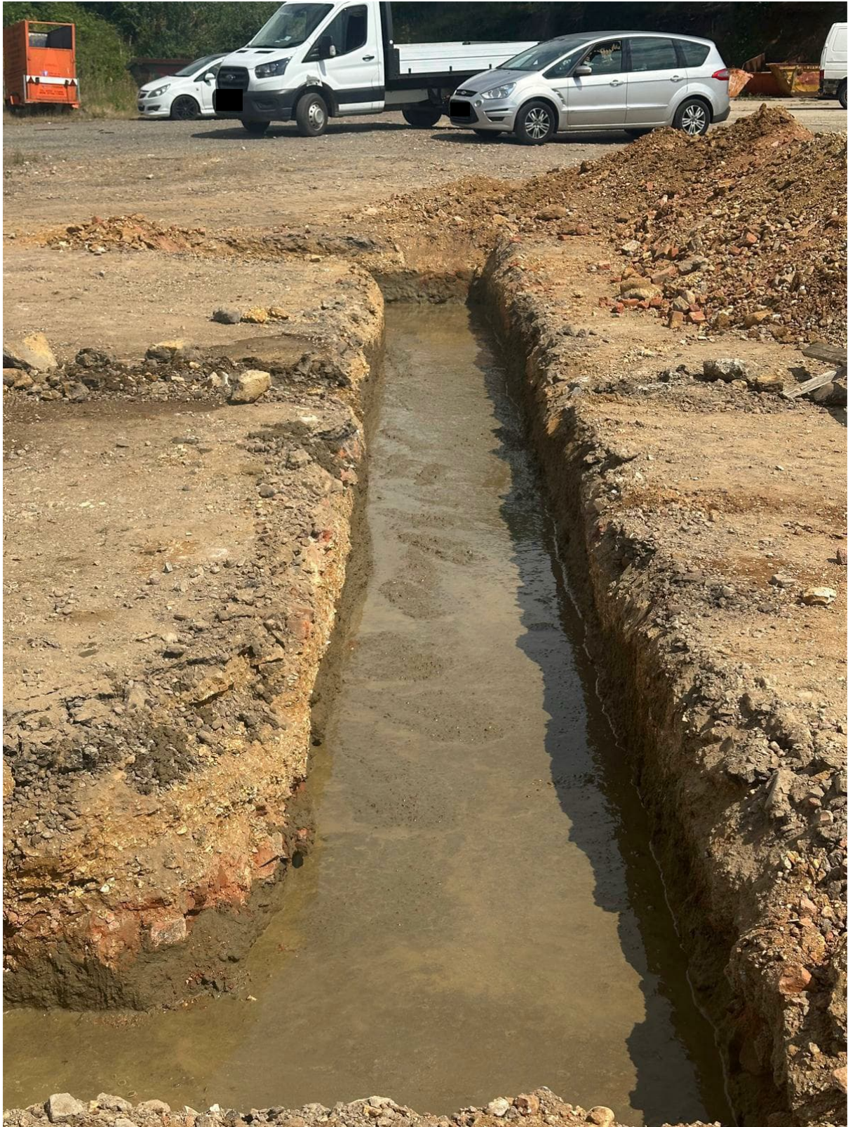
21/01535/F - Vicars Grove Pit, Little Almshoe Road, St Ippolyts, Hertfordshire: Evidence of a Material Start on Site
