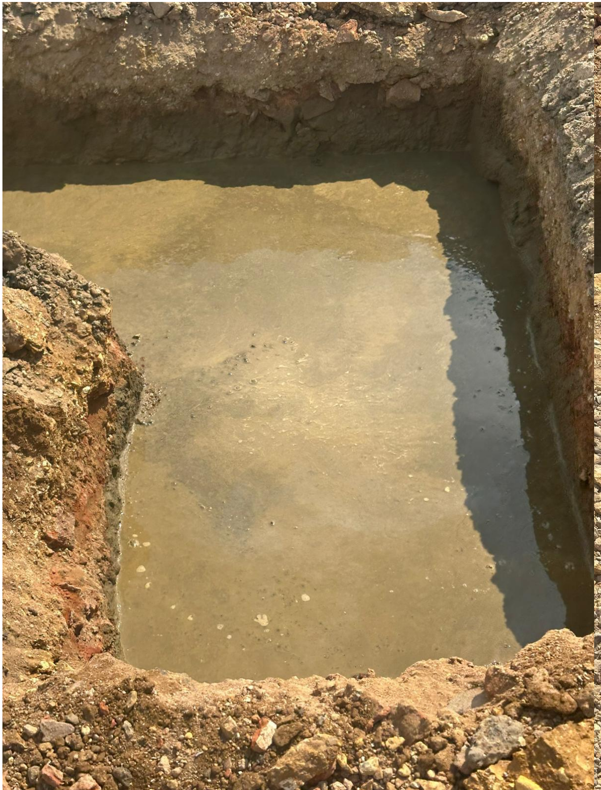
21/01535/F - Vicars Grove Pit, Little Almshoe Road, St Ippolyts, Hertfordshire: Evidence of a Material Start on Site
