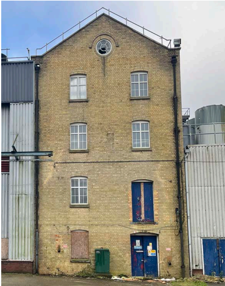
Full front elevation of the existing mill
