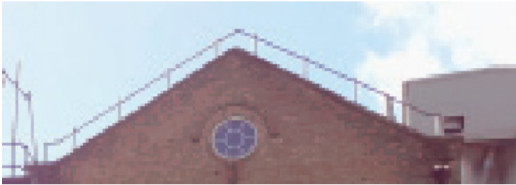
Roof detailing on gables
