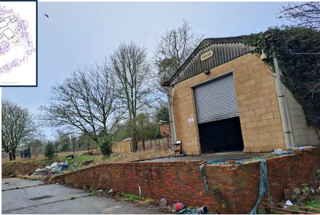
Photo 1 of the northern boundary, looking north east. All photos taken 16 January 2026 unless otherwise stated.
