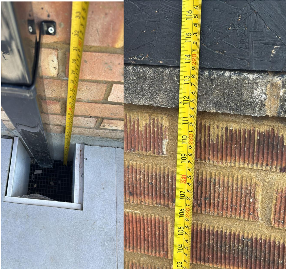
3m from ground level to flat roof
