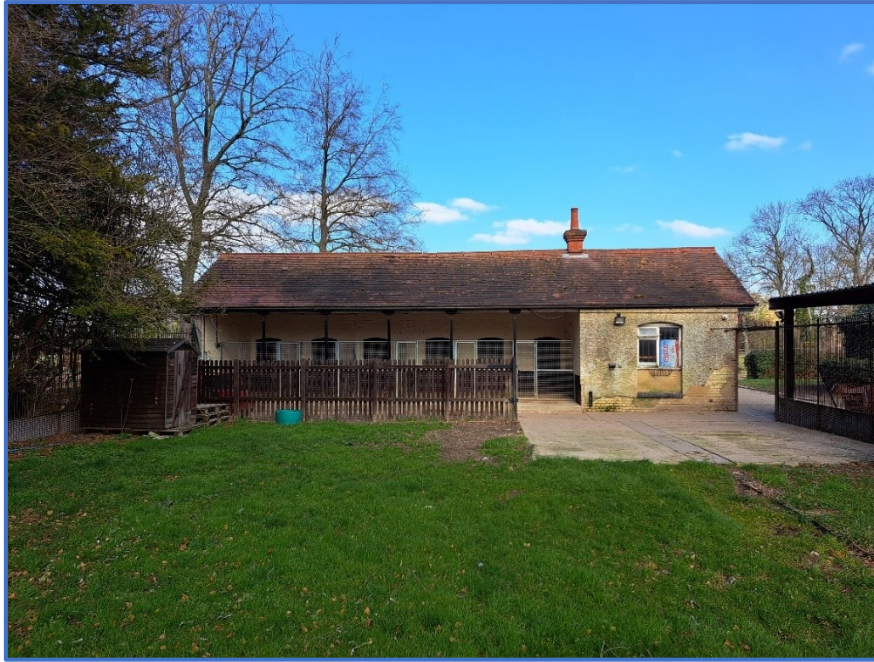
Figure 3 – View of rear elevation of Kennels building
