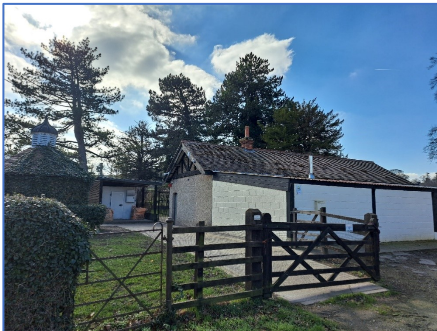
Figure 2 – View of front elevation of Kennels building
