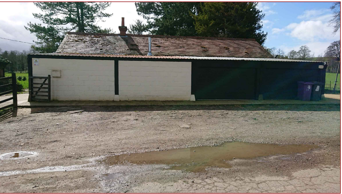
Existing Kennel Image (North)
