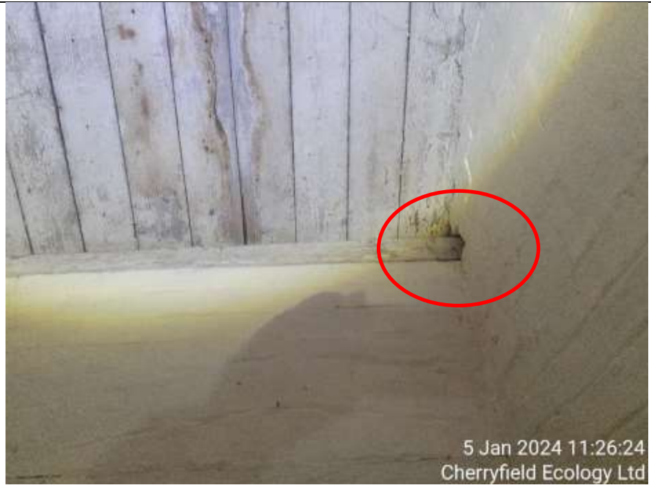
Figure 8: further example of gap in the open access area
