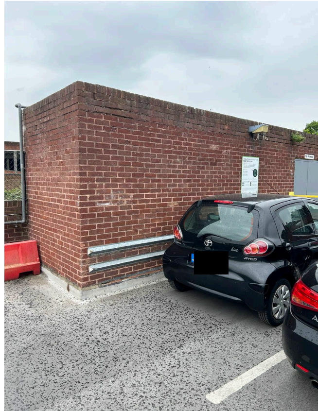
Photograph 5: Brick structure / outbuilding situated in the car park (according to aerial imagery this appears to be along the southern site boundary).
