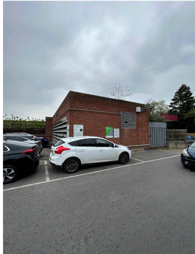
Photograph 2: Loading Bay Area Facing West
