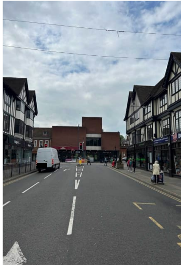
The Stop End to Hermitage Rd
