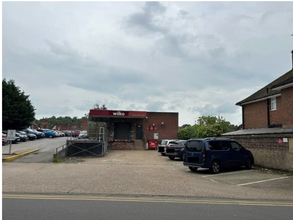
Grammar School Walk Parking and Servicing Access
