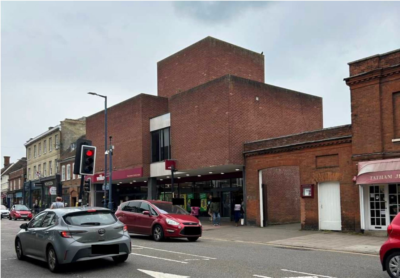
Photograph 03 - Stood outside No. 110 Bancroft Looking West
