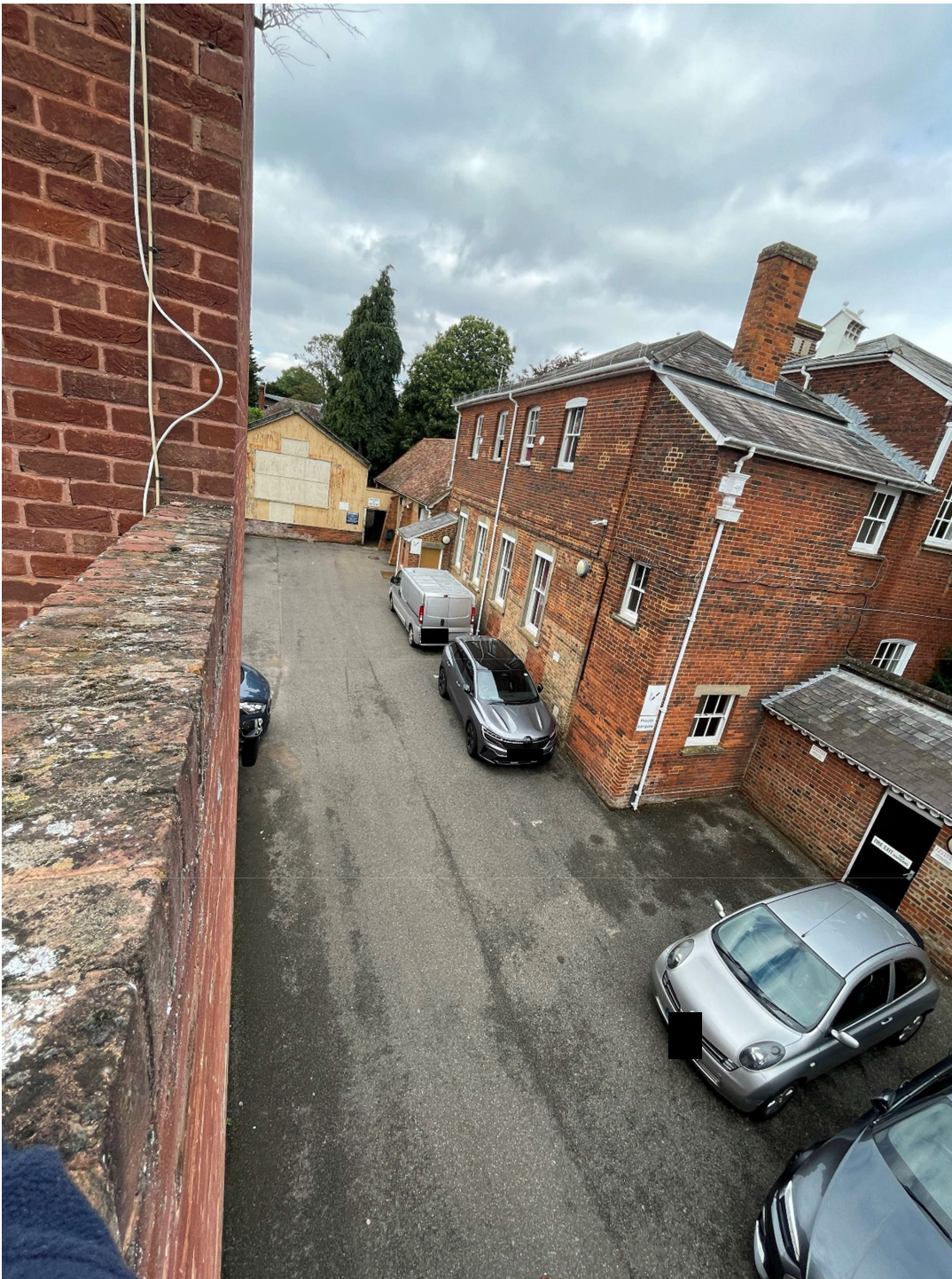
Photograph 14 - At Carpark level looking North West towards 20 Bancroft & The Grammer School
