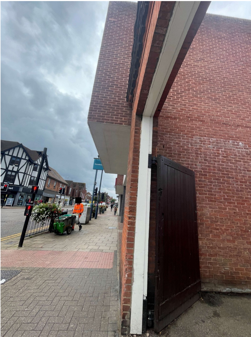
Photograph 06 - Stood to the right of site Looking South towards The existing side elevation
