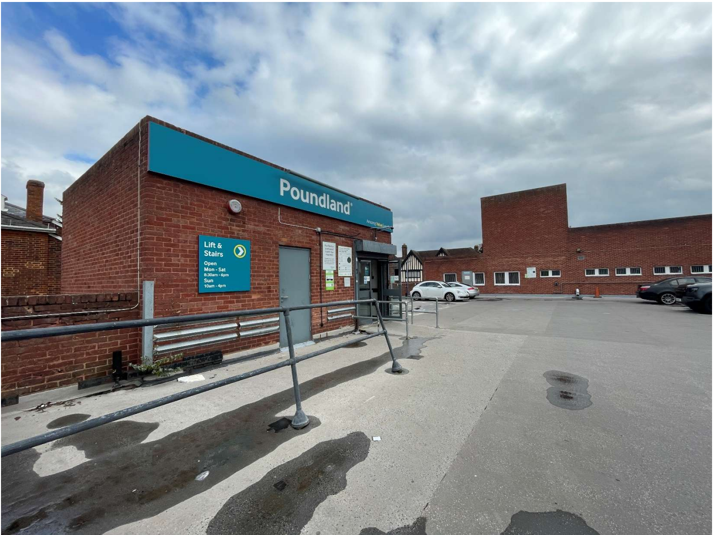
Photograph 18 - At Carpark level looking East towards the staircase to Poundland store level and the rear of 18-19 Bancroft
