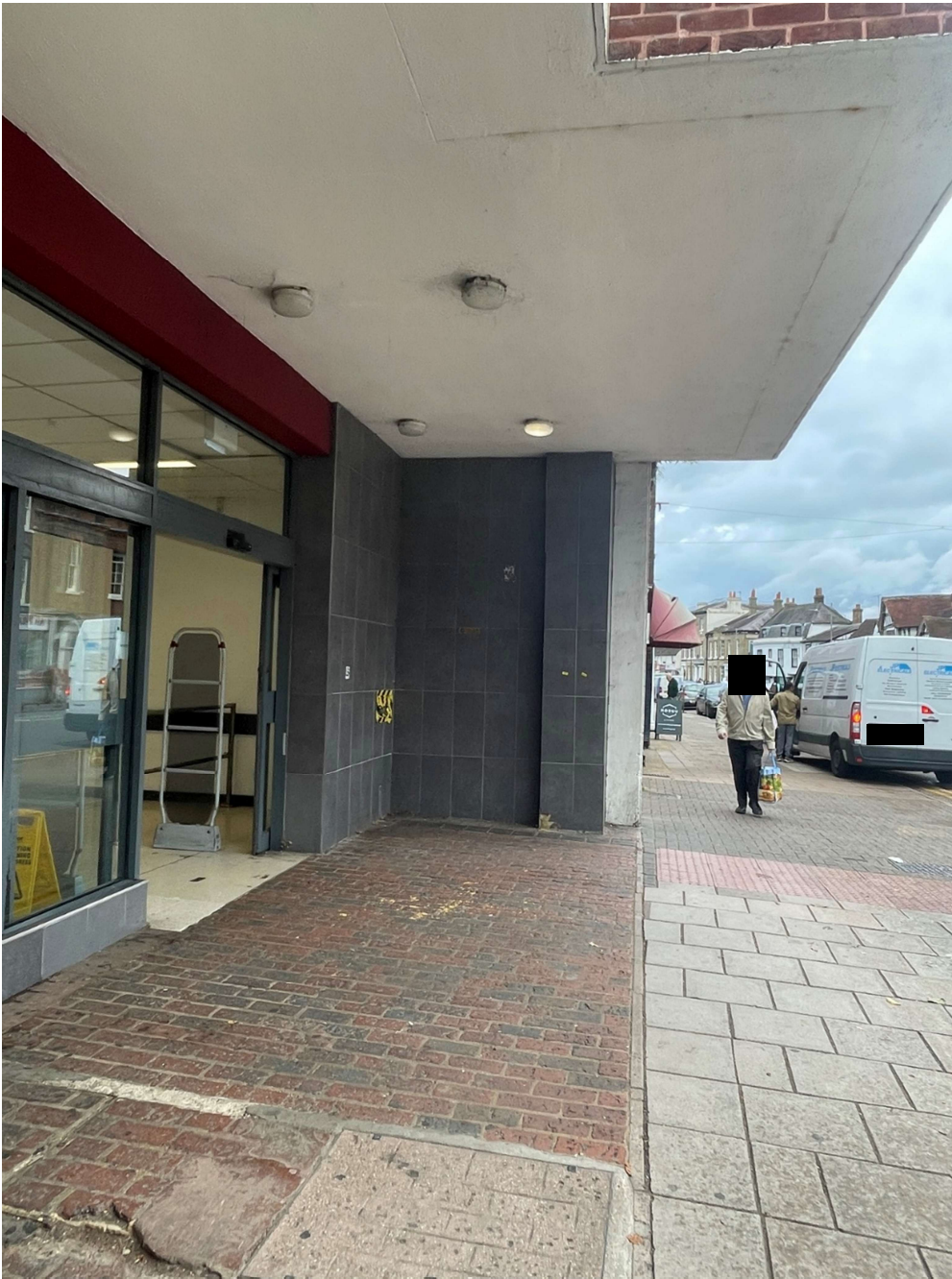
Photograph 05 - Stood under the overhanging first floor looking North
