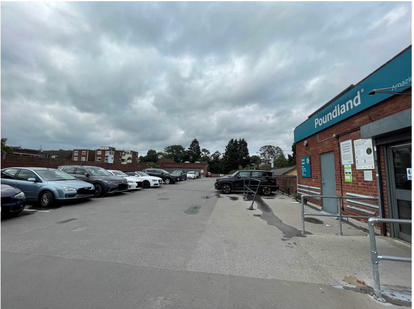
Photograph 16 - At Carpark level looking North West towards Grammar School Walk & the rear of Netherwood
