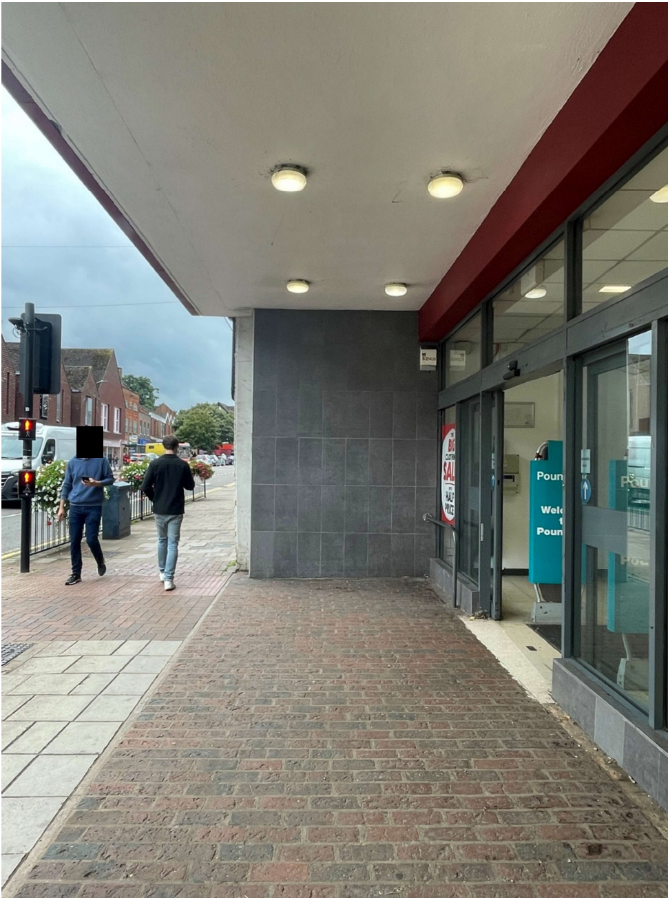
Photograph 04 - Stood under the overhanging first floor looking South
