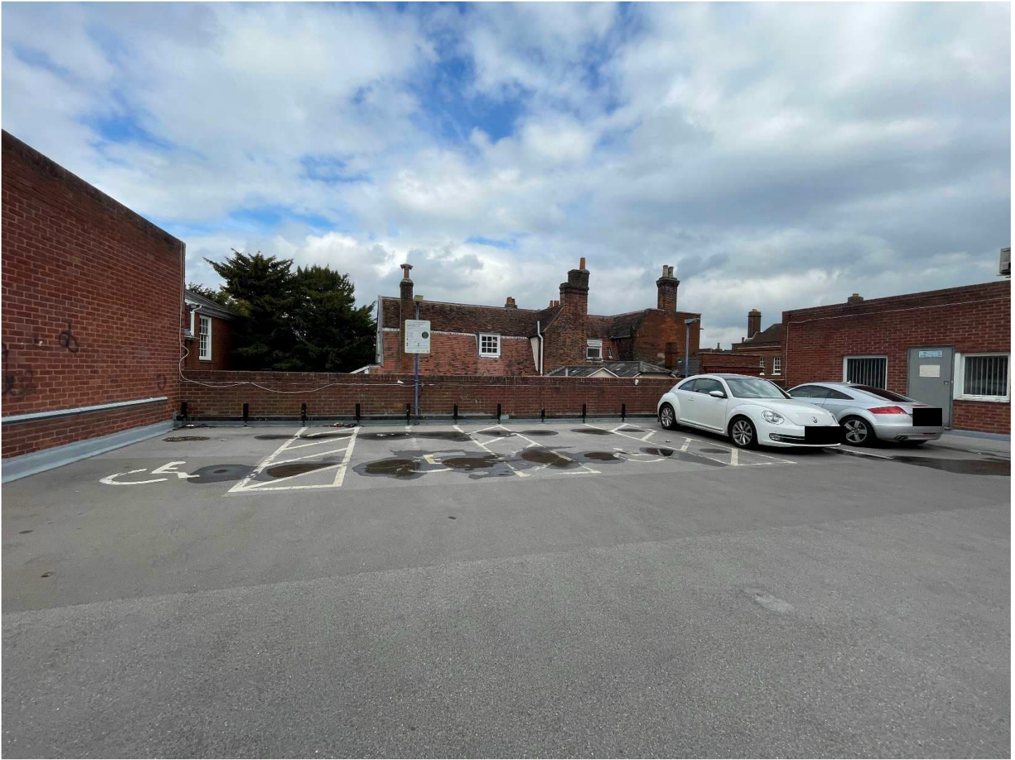
Photograph 15 - At Carpark level looking North towards 20 Bancroft
