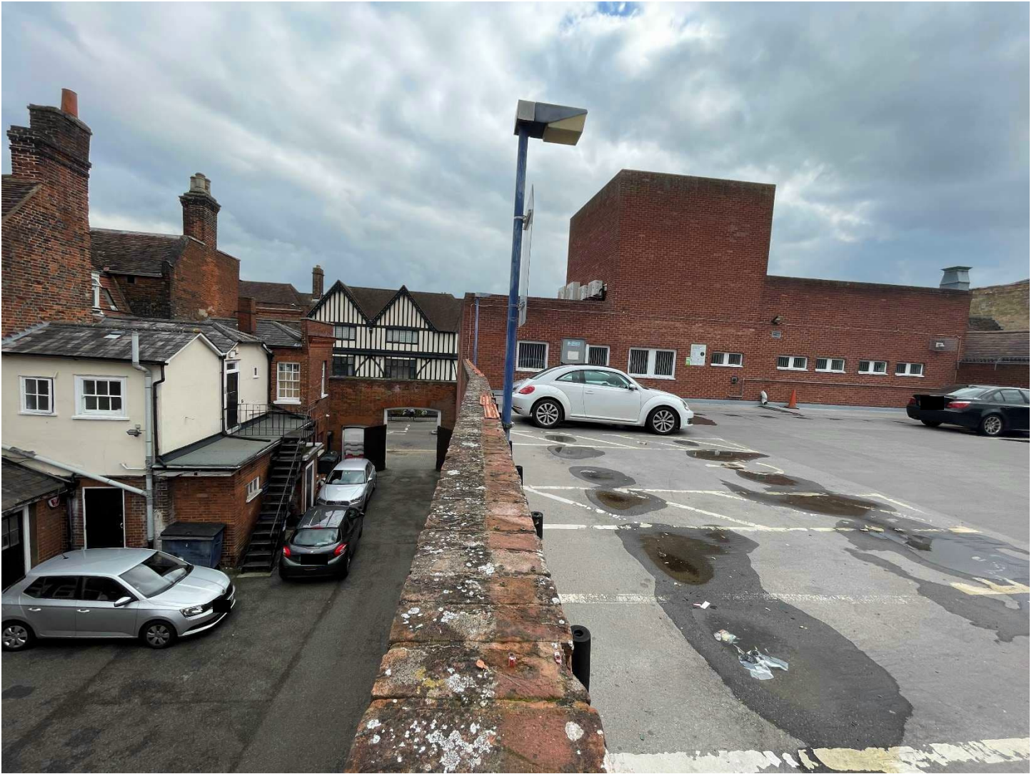
Photograph 13 - At Carpark level looking East towards 112 Bancroft
