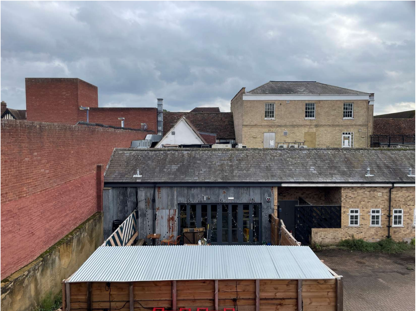
Photograph 17 - At Carpark level looking South East towards the rear of 15-17 Bancroft
