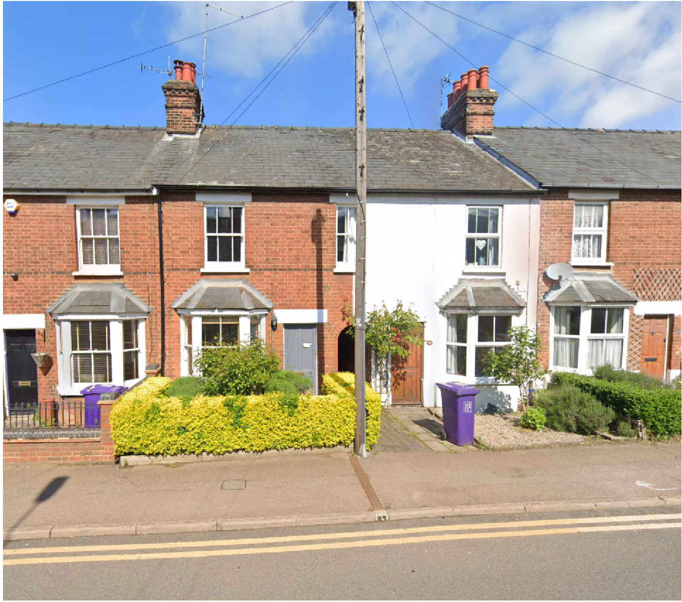
FRONT VIEW OF EXISTING PROPERTY
