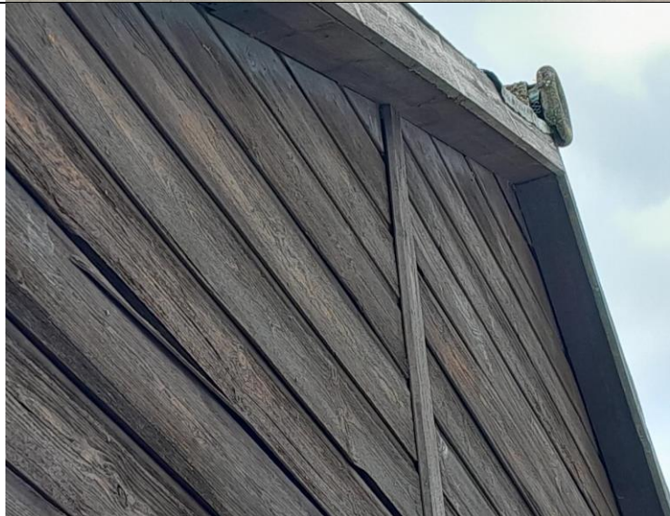
Figure 3 – lifted bargeboard on western end of B1
