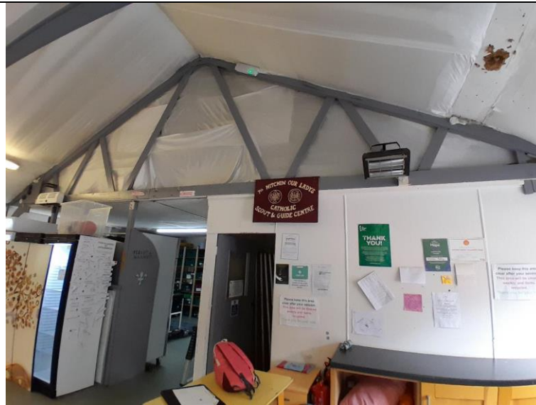
Figure 10 – interior of mezzanine loft space in B1
