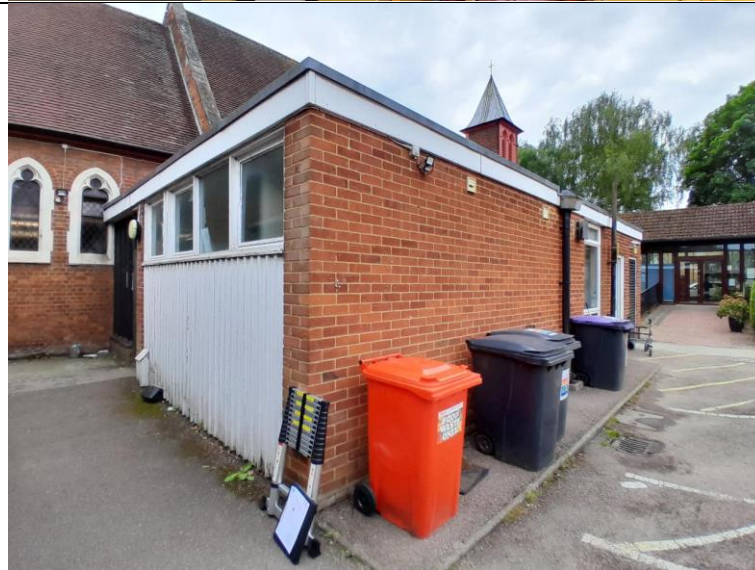
Figure 12 – southern and western elevation of B2
