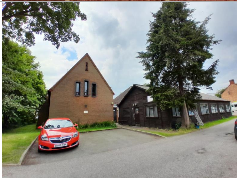
Figure 16 – hardstanding area at the centre of the site, to the southeast of B1
