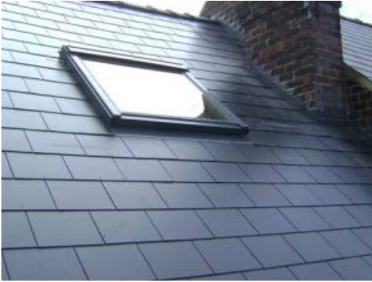
(man made slate roof tiles precedent)
