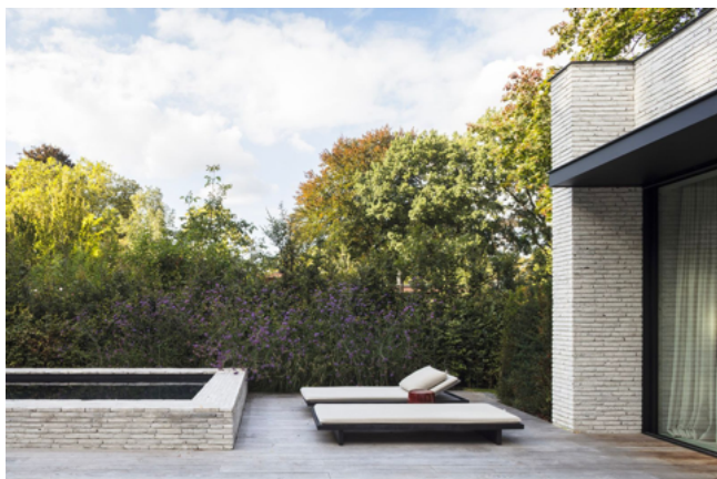
Retaining walls & swimming pool / Chalk long brick
