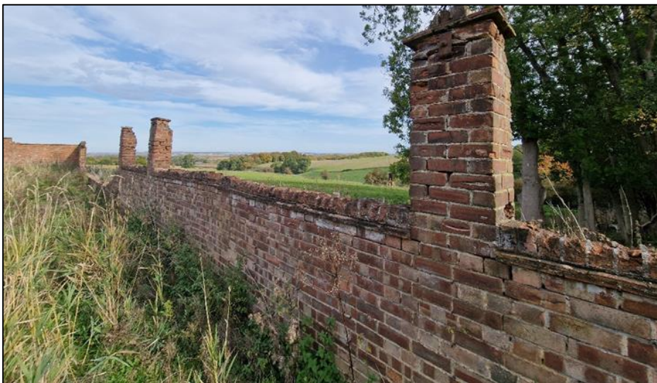
Plate 9: part of the southeastern boundary wall looking northeast from the interior of the garden
