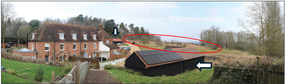
Plate 13: view of the walled garden (ringed) relative to the Dower House (centre left); recent modern interventions to outbuildings are arrowed
