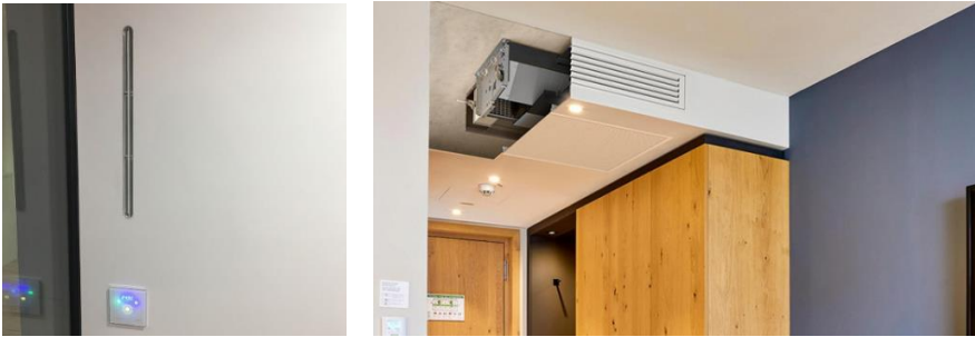
Figure 10: Example of cooling wall vent and thermostat (right) and ceiling fan coil unit (left)
