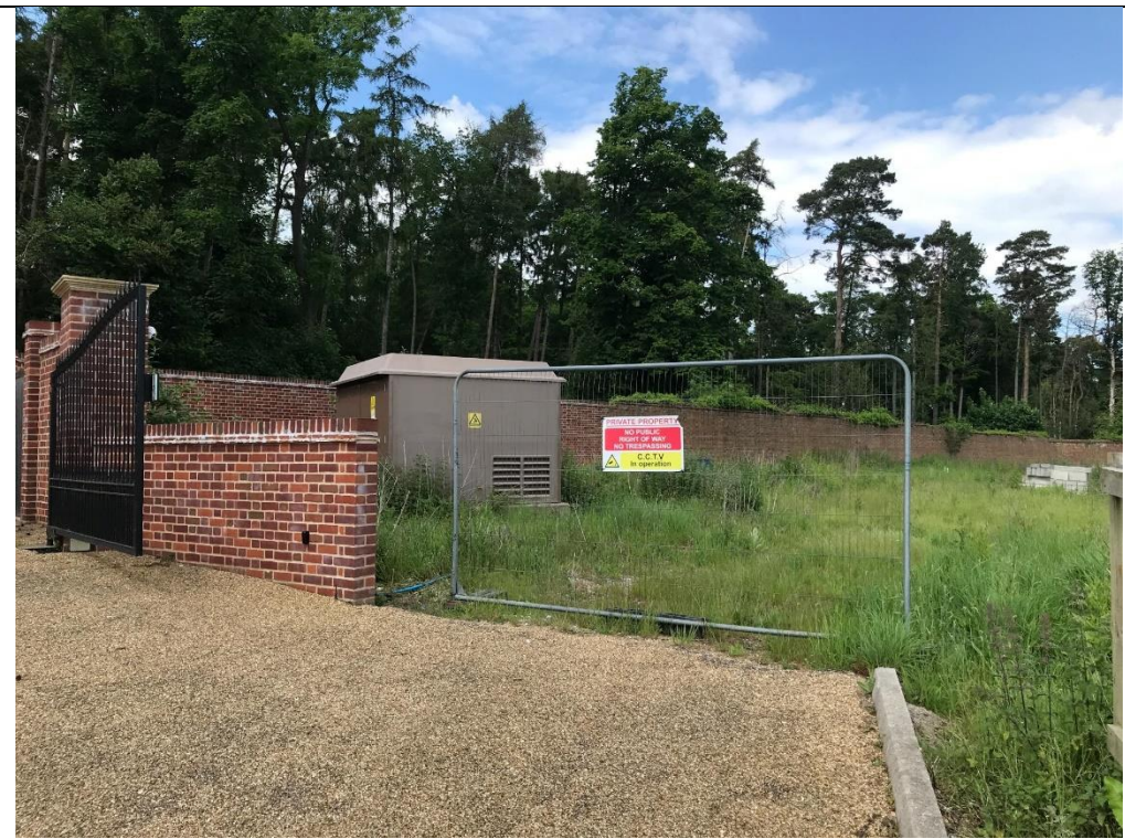
Plate 6: Facing into the site. Existing substation visible in left hand side of this image.
