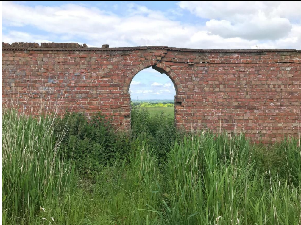
Plate 11: An entrance within the northwestern part of the former walled garden.
