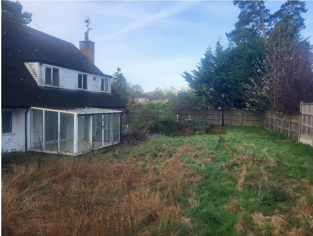
Photo 3 – Area to rear of the property with restricted access
