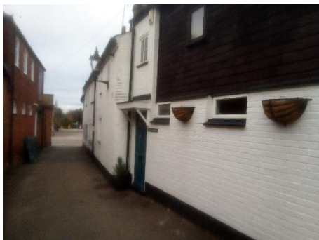
Walnut Cottage, Bakers Lane
