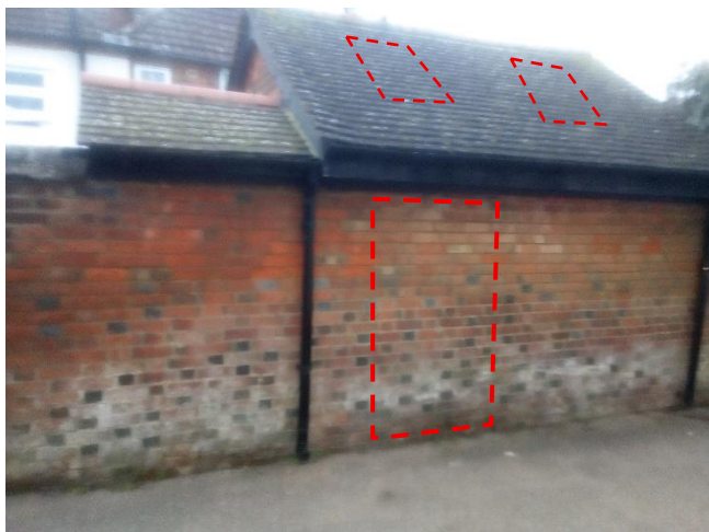
Existing rear elevation of the property.
