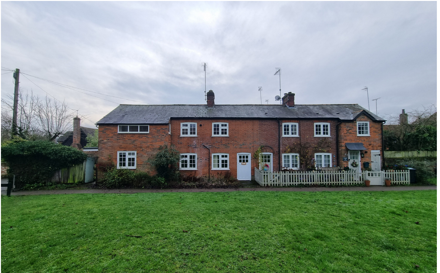
Above: Elevation of 19 and 20 Garden Fields from Garden Fields with number 19 being on the left hand side with the fenced garden.
