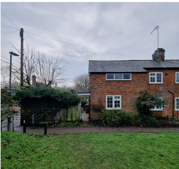
Existing 19 Garden Fields garden entry gate
