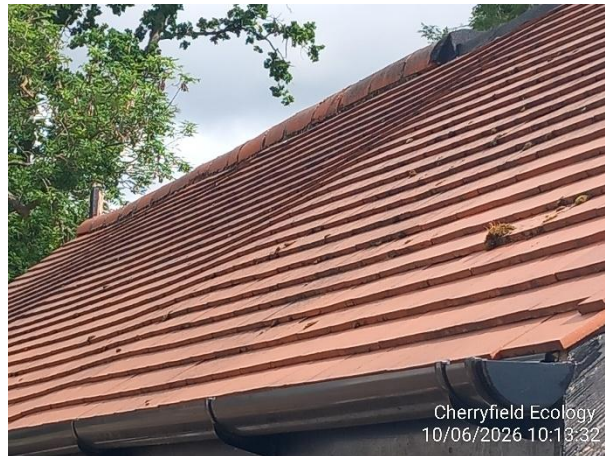
Figure 7: Example of the roofing tiles, including some of the felt on the ridge line
