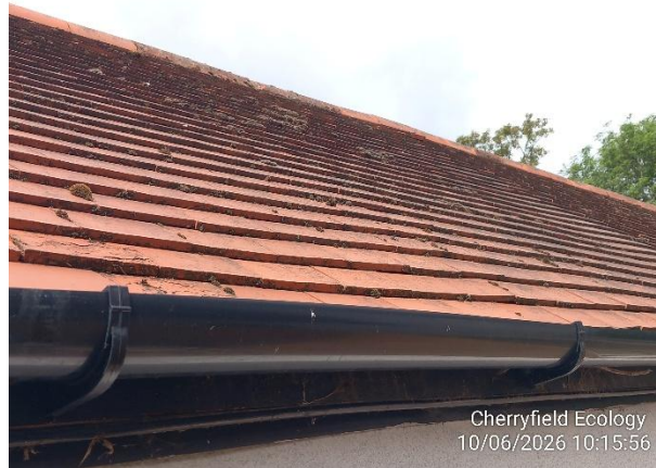
Figure 6: Example of the roofing tiles
