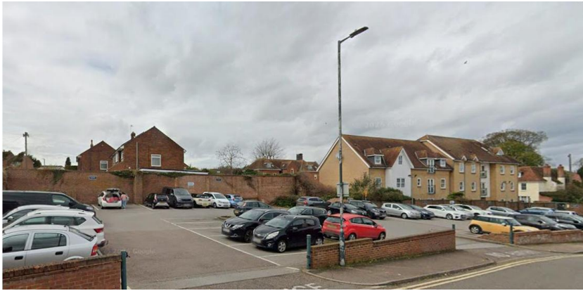
Existing car park
