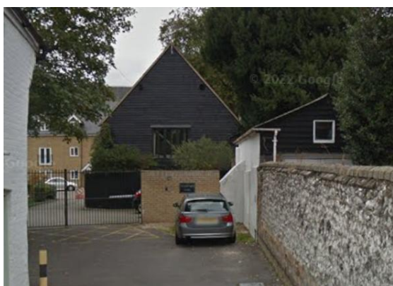
Ancillary buildings, rear no 8 Lower King Street
