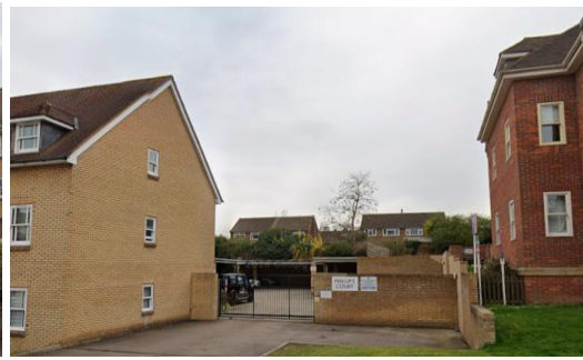
2. View from Baldock Street
