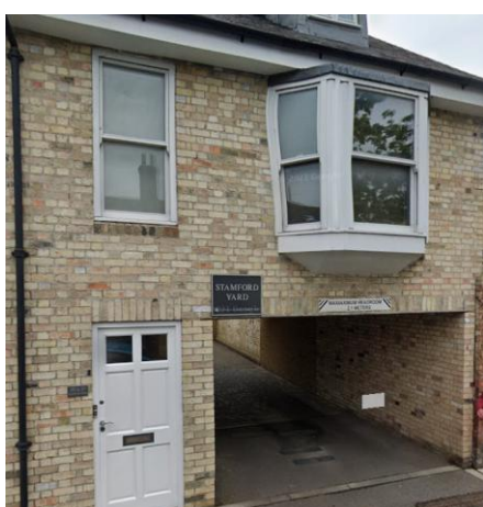
Stamford Yard, Lower King Street
