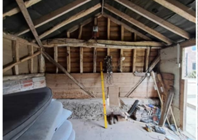
Structural Truss & Central partition
