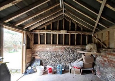
Structural Truss & Central partition
