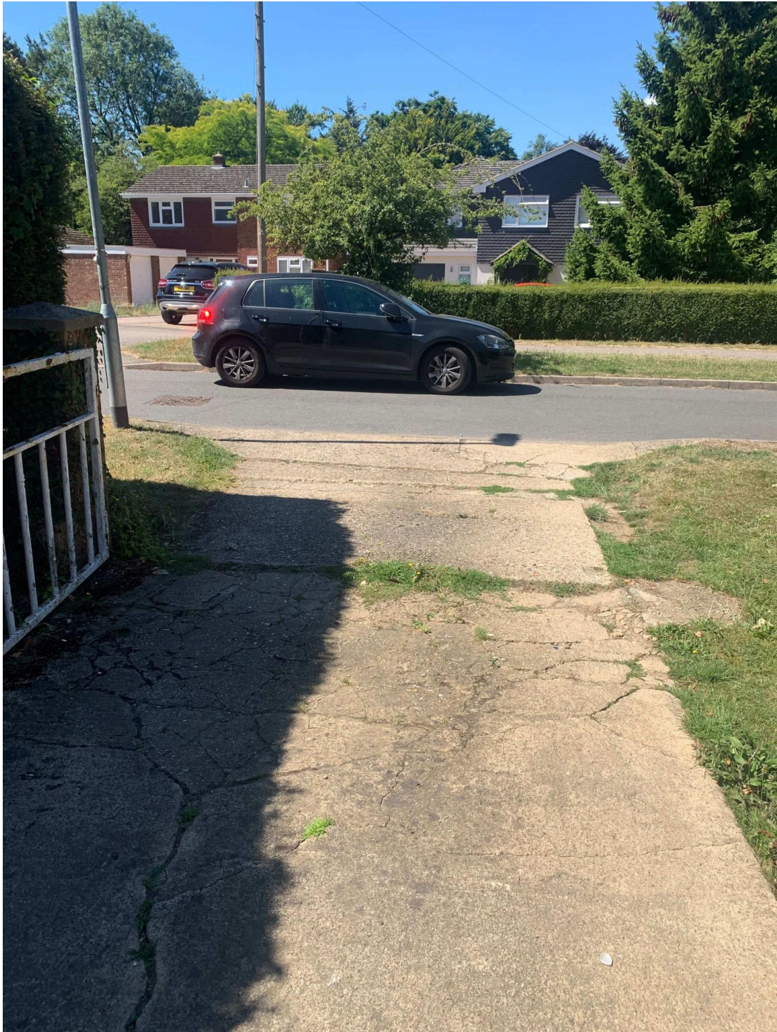
Photograph 16: 14 Cashio Lane prior to the works — the original single gate opening onto the concrete driveway. This is the pre-works access arrangement referred to in paragraph 2.3.
