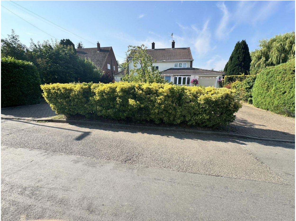
Photograph 20 — 22 Croft Lane: Clear dual crossover arrangement at 22 Croft Lane — two wide dropped kerb access points either side of a central hedge island, in an identical concept to the appellant's turning circle arrangement. No footpath present. This arrangement is long-established and has not been subject to enforcement action.
