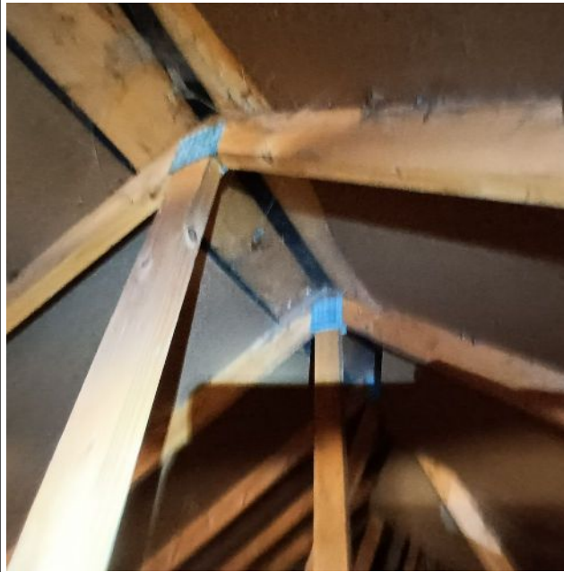
Figure 9: View of ridge beam and lining
