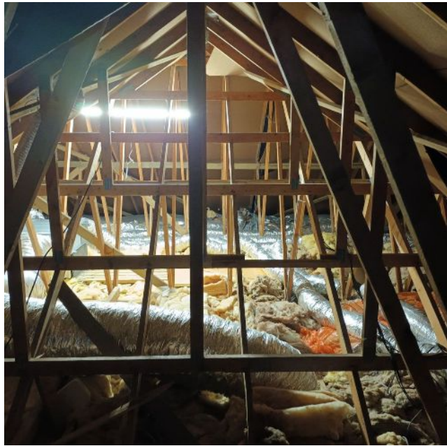
Figure 8: View of loft from north end looking south
