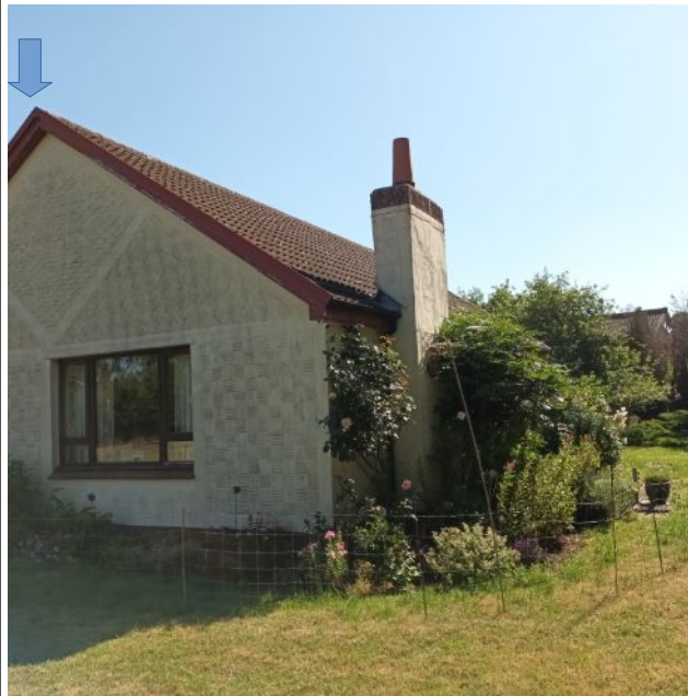
Figure 6: View of western gable Bat roost is located at arrow
