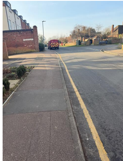
Photograph 3: Existing conditions of Wratten Road East
