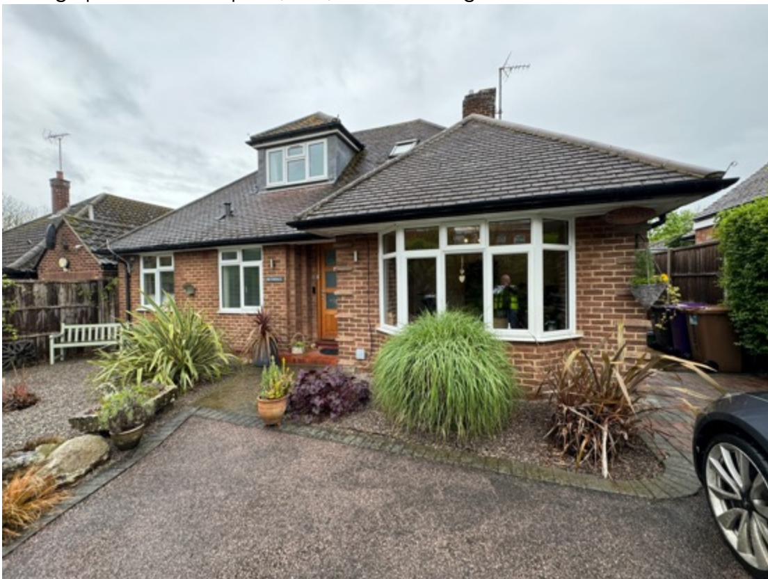
Photograph 6: Eastern aspect (front) of the dwelling at Silverdale
