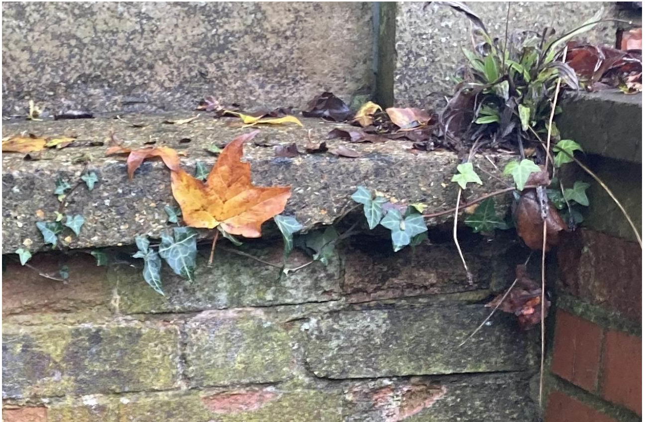
16. The brick plinth has a number of bricks with spalled faces.
