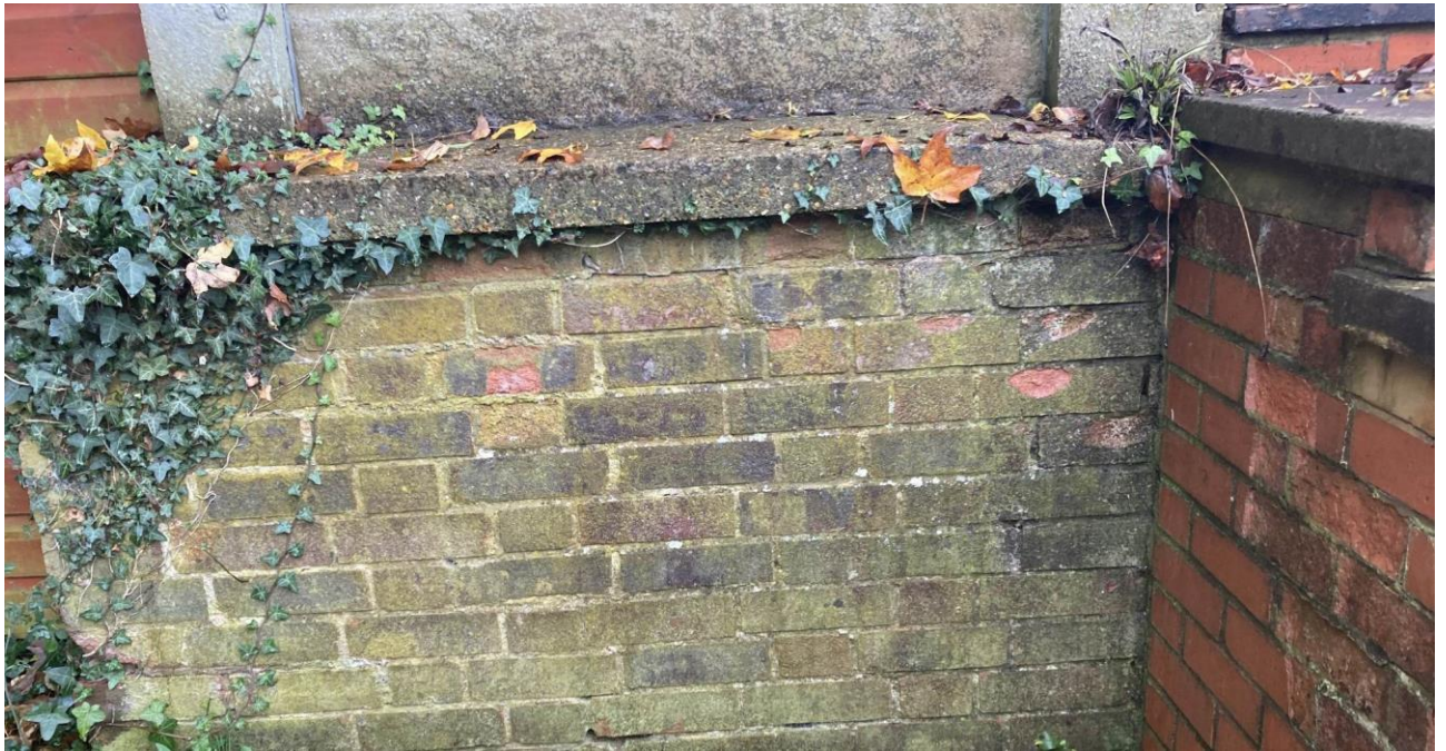
16. The brick plinth has a number of bricks with spalled faces.
