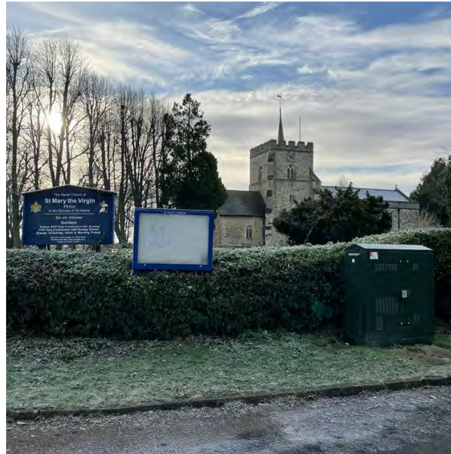
Fig.15: St. Mary's Church: A Grade I listed building
