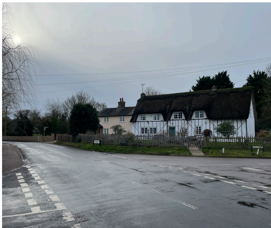
Figure 4.6 4 - 6 Walnut Tree Road (Grade: II, List Entry Number: 1347097)
