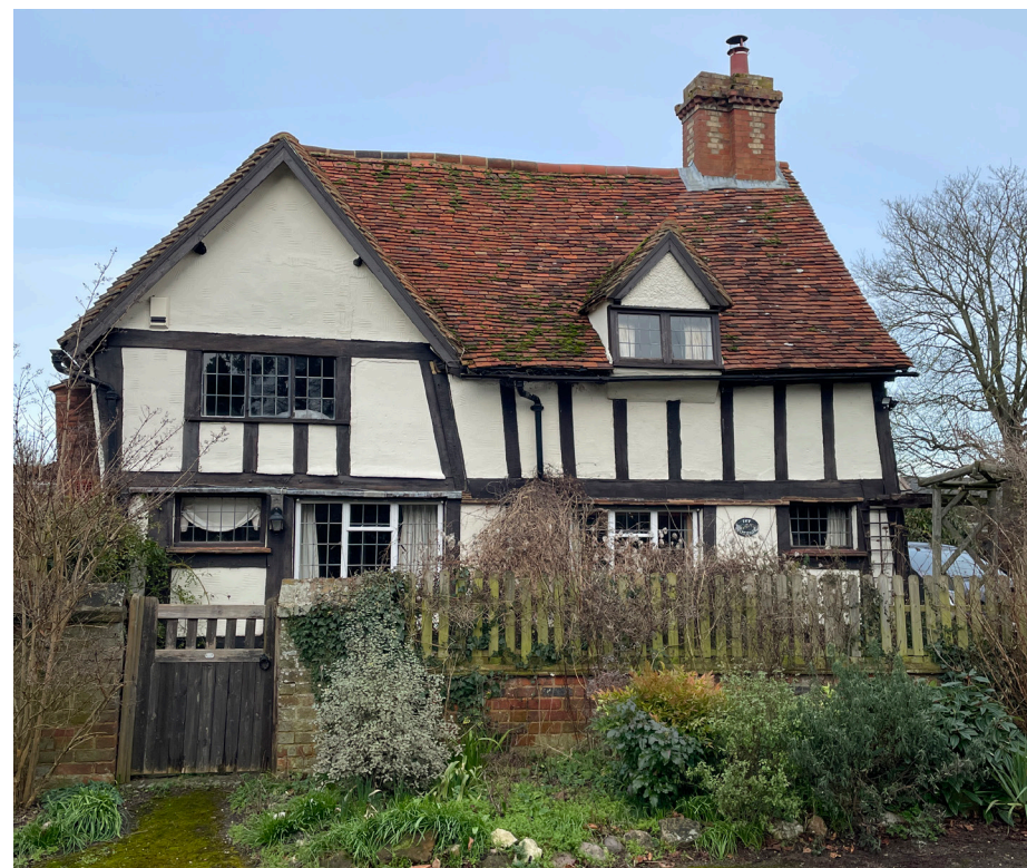
Figure 4.7 Ivy Cottage (Grade II, List Entry Number: 1103187)
