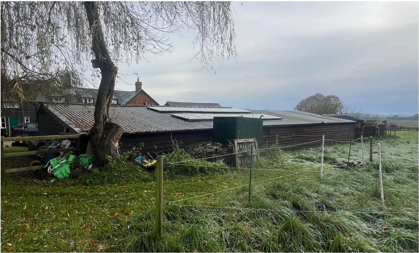
2. Existing view of rear
