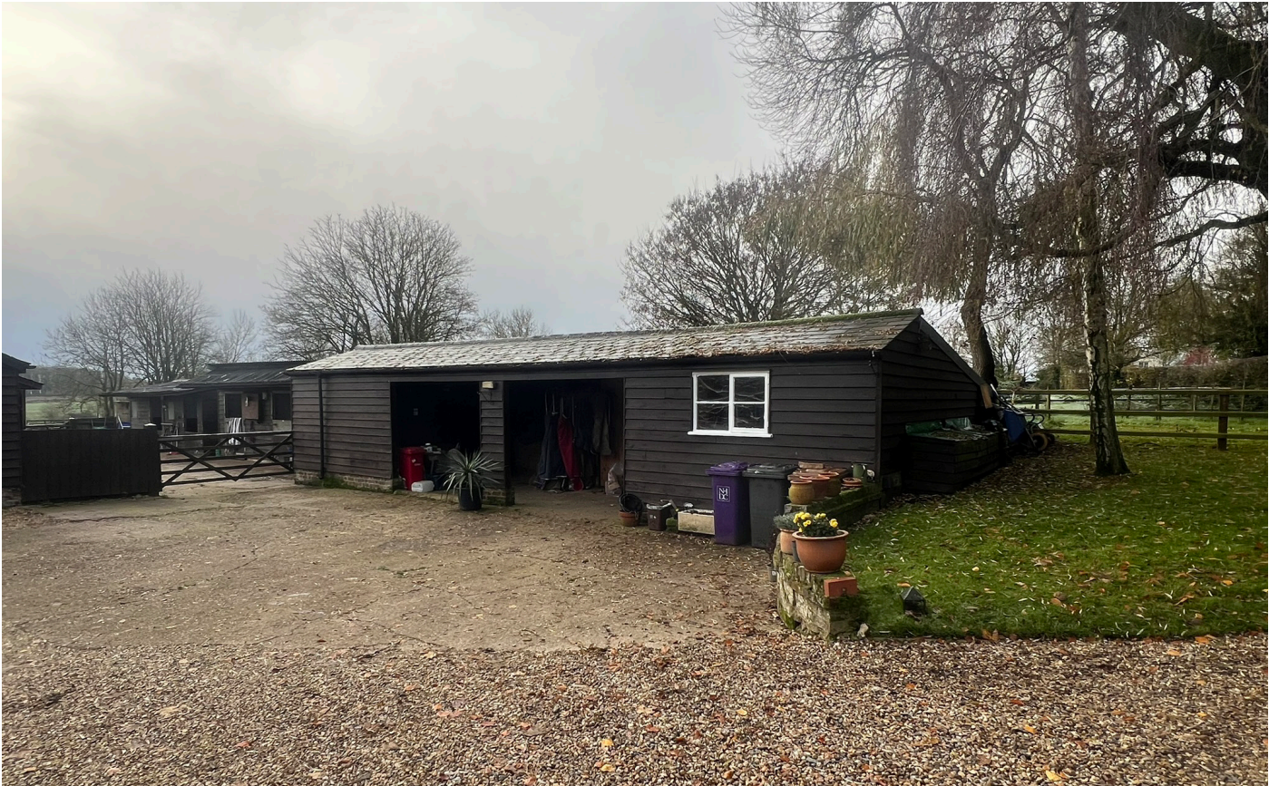
1. Existing view of front
