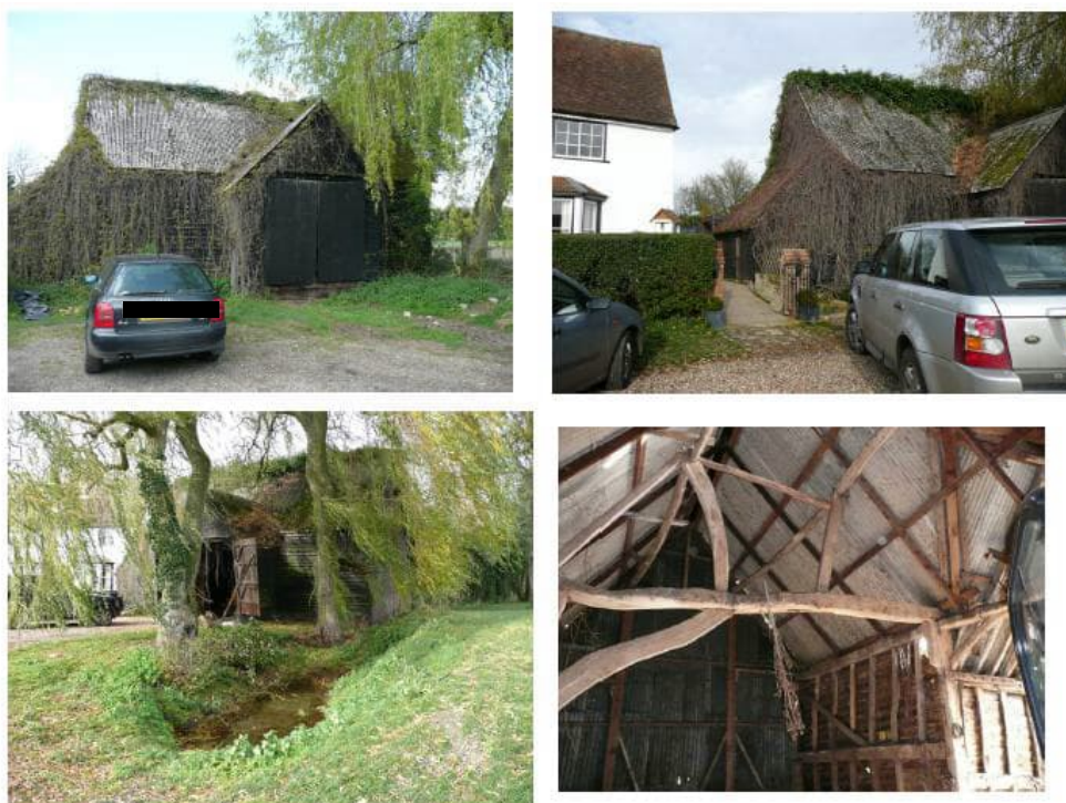
Figure 2 - Photographs of the barn from application ref. 25/00509/FPH
