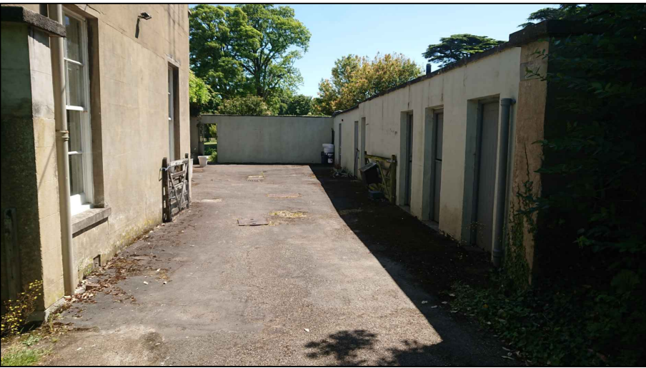
Photograph of Front of Service Building
