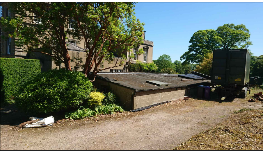
Photograph of Rear of Service Building
