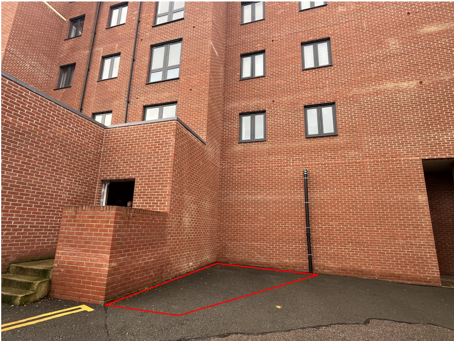
Photo of rear elevation of building showing Plant location
