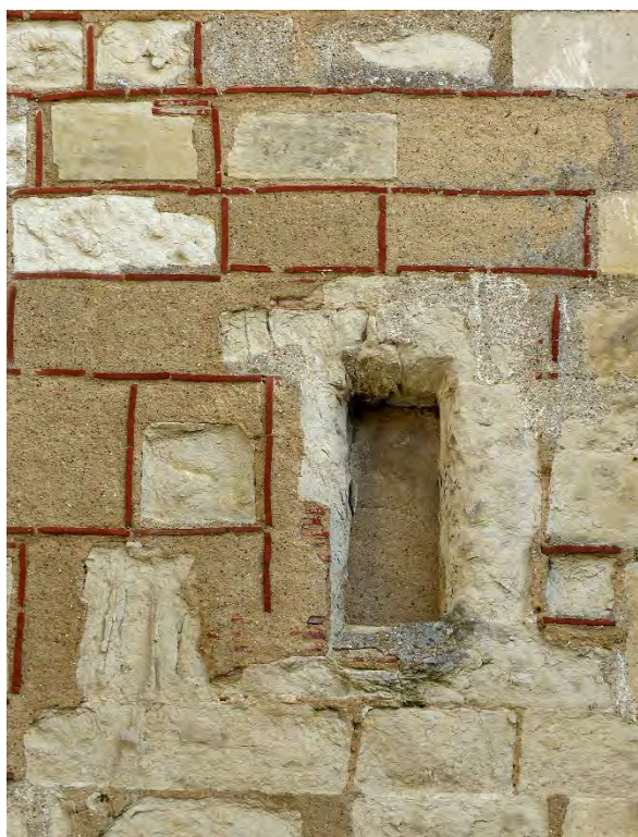
Fig. 49 (left). Tile and render repairs on the west wall of the south porch, an example of Weir's work.
