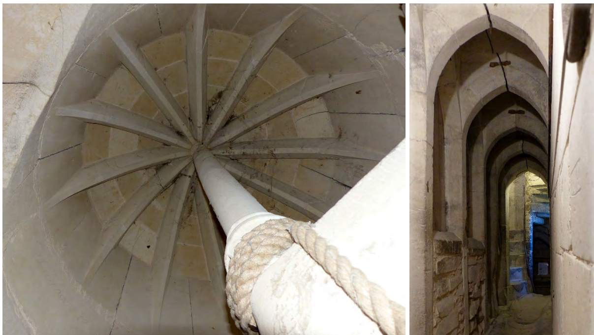
Fig. 9 (left). The vault at the top of the south-west stair.
