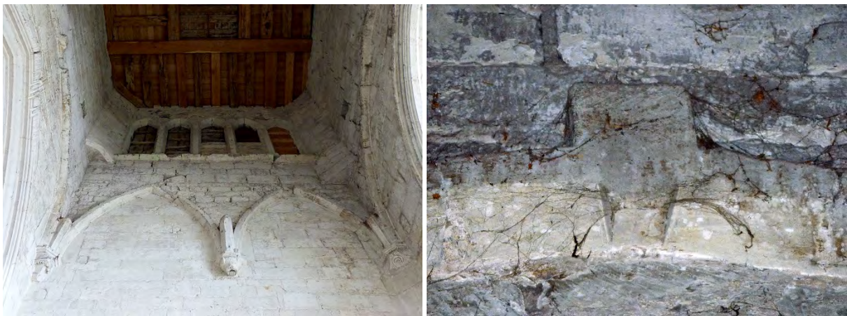
Fig 7 (left). Remains of the vault, with the gallery arcade above, viewed from the north.
