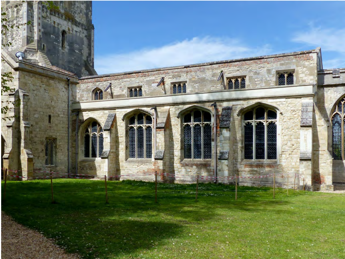
Fig. 18. Bays 3 to 6 of the south aisle and 2 to 6 of the clerestorey
