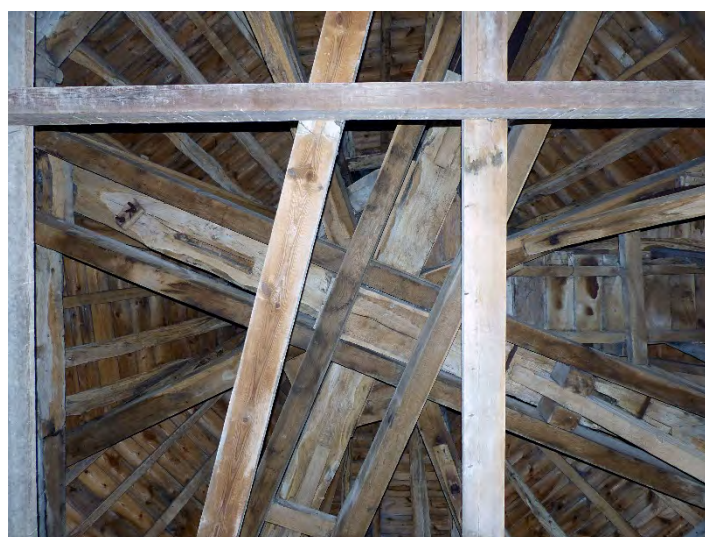
Fig. 17 (right). The base of the spike, seen from the fourth stage below. The principal beams form a cross, and lesser beams bisect the angles between them. Braces originally rose from the frame below to all eight beams.
