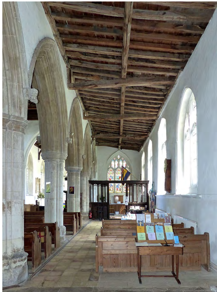
Fig. 24 Interior of south aisle, looking east towards the Lady Chapel (with later parclose screen).
