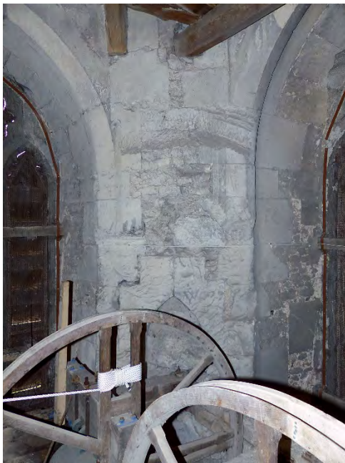
Fig. 13 (left). Interior of belfry, showing blocked doorway in south-east corner, indicated by pointed two-centred arch low down, its crown just above the further wheel.
