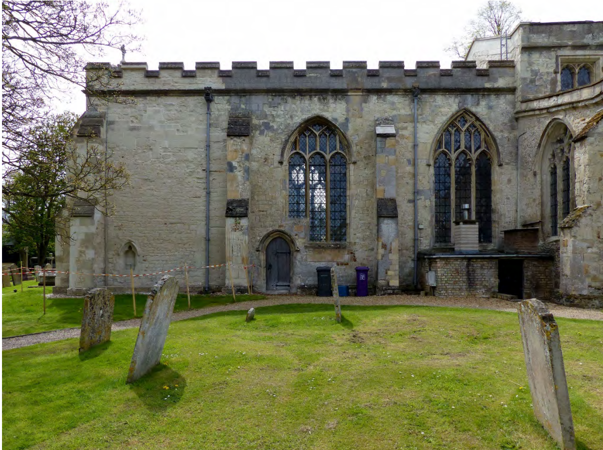
Fig. 30. The north elevation of the chancel, showing the blind eastern bay incorporating a blocked doorway to the demolished vestry, and a niche for a holy water stoup. The priest's doorway occupies the central bay.
