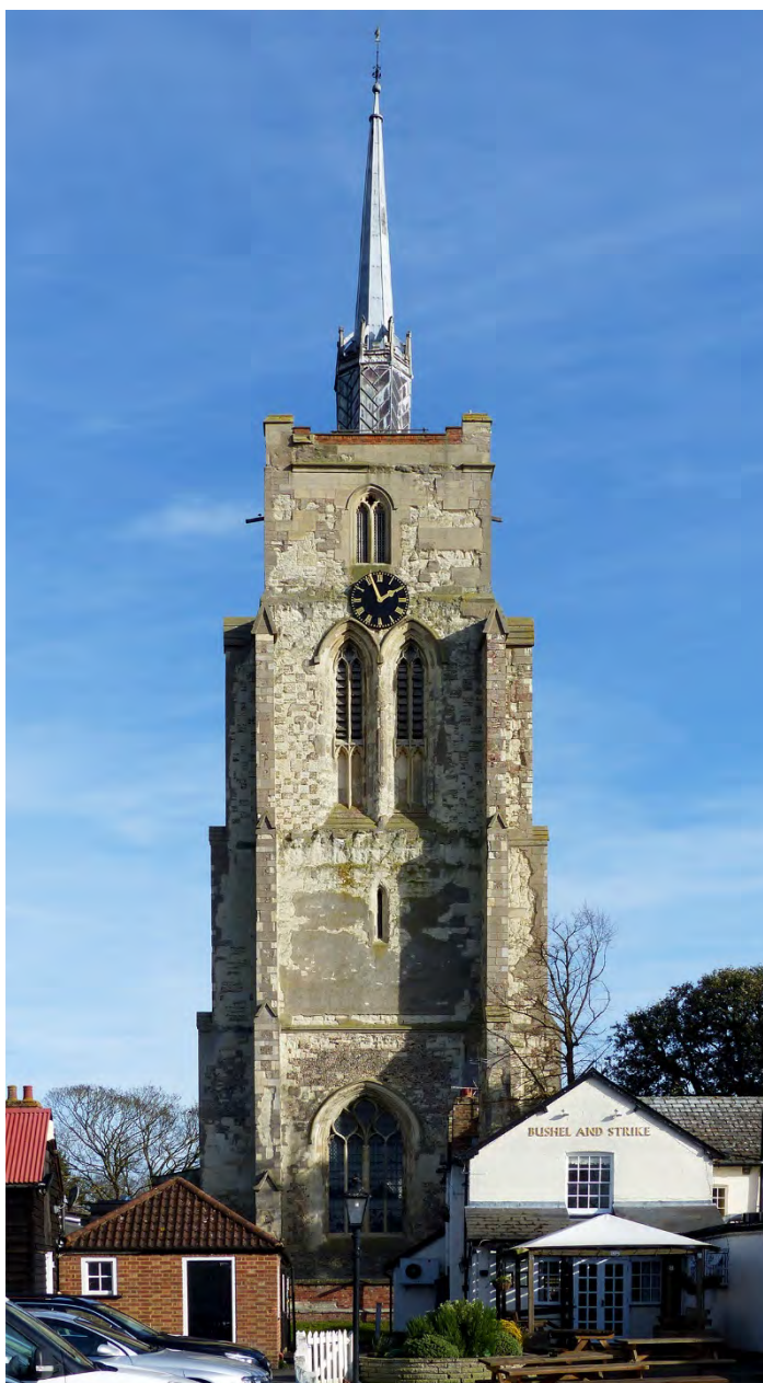
Fig. 4. The west elevation of the tower
