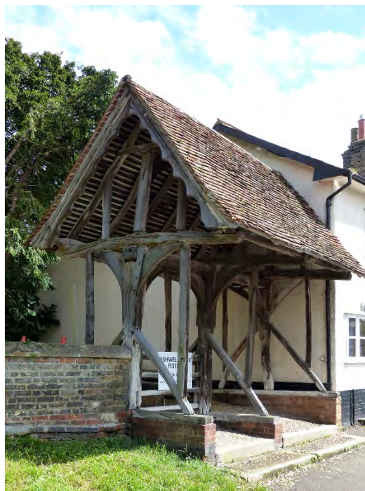
Fig. 61. Lychgate from the north-west.
