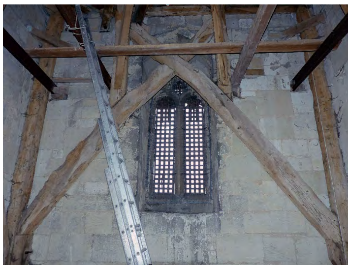
Fig. 15. Wall-posts and scissor-braces with struts rising from the latter just below the halving joint.
