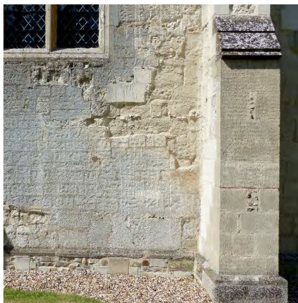
Fig. 49 (left). Tile and render repairs on the west wall of the south porch, an example of Weir's work.
